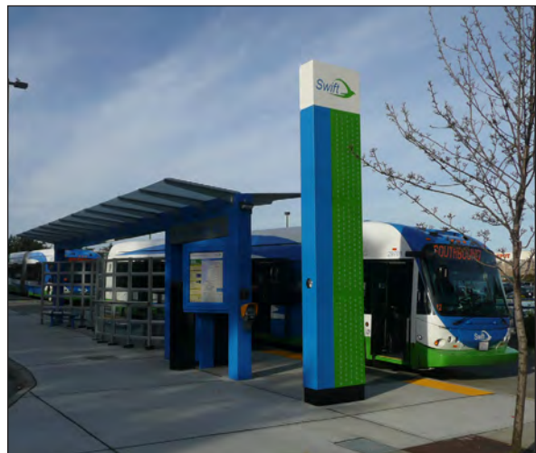
Swift station on SR 99
