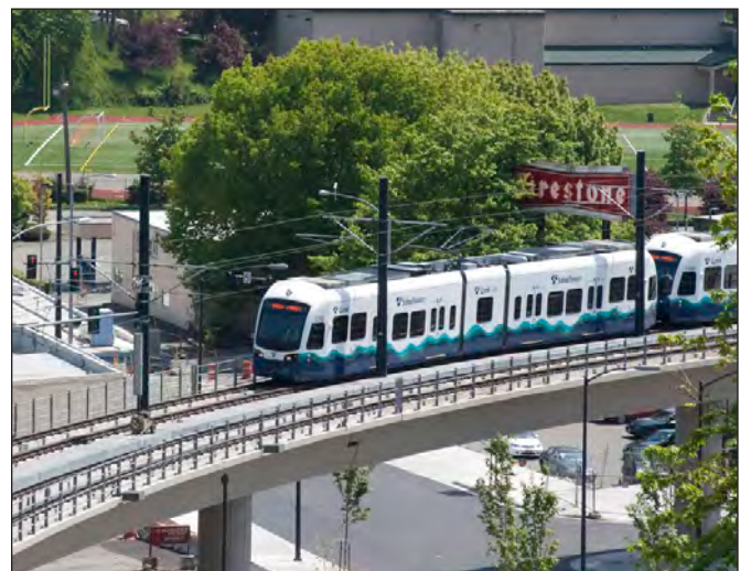
Elevated light rail
