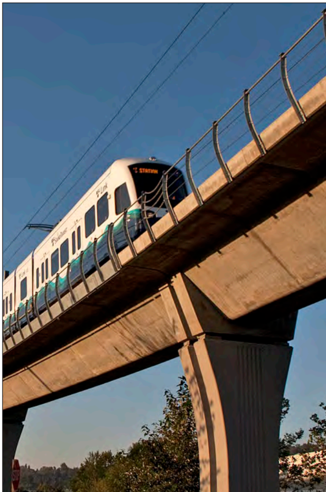
Elevated light rail
