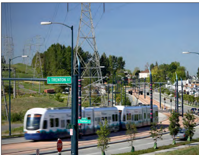
At-grade light rail at South Trenton Street
