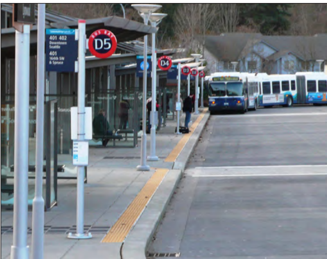
Existing Lynnwood Transit Center
