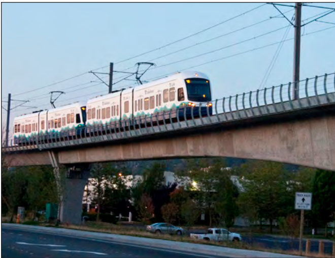
Elevated light rail
