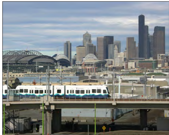
Link Light Rail in downtown Seattle
