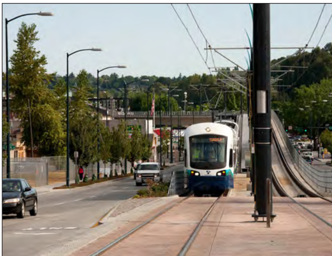
Light rail transitions from elevated to at-grade
