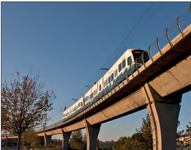
Elevated light rail
