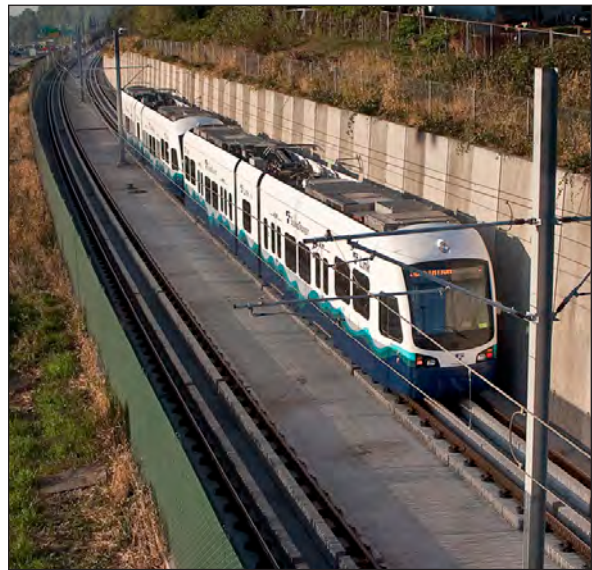
Light rail in retained cut
