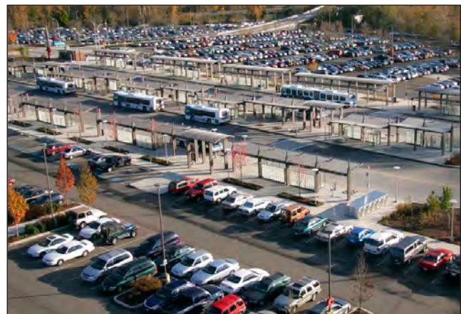
Lynnwood Transit Center
