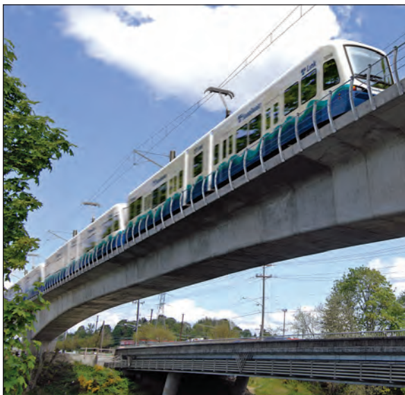
Elevated light rail
