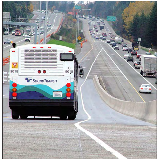
I-5 HOV direct access ramp in Lynnwood
