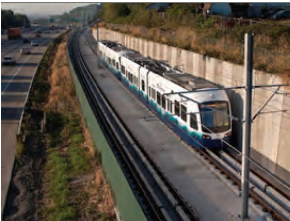
At-grade Light Rail Train
