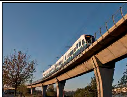
Light Rail Train with Overhead Catenary Wires in Tukwila, WA
