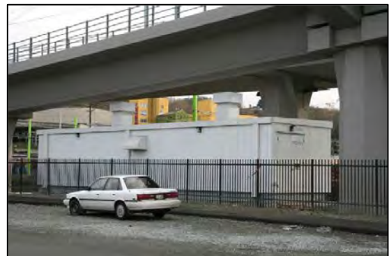
Example of a Traction Power Substation
