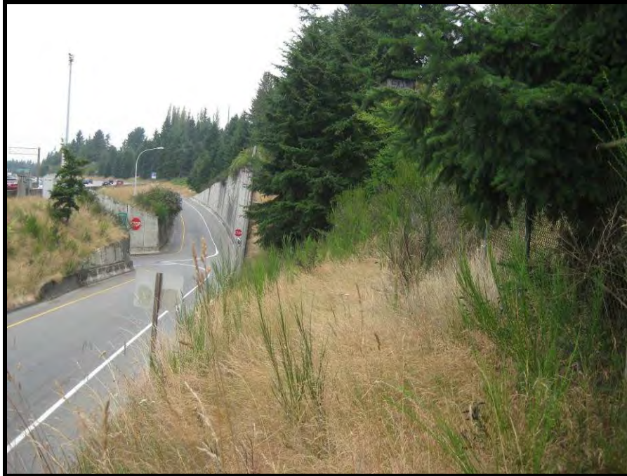
Figure 2-2. Overview of I-5 APE/right-of-way in Area 11, view north
