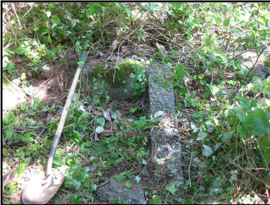
Figure 3-4. Overview of remnant concrete foundation, view north
