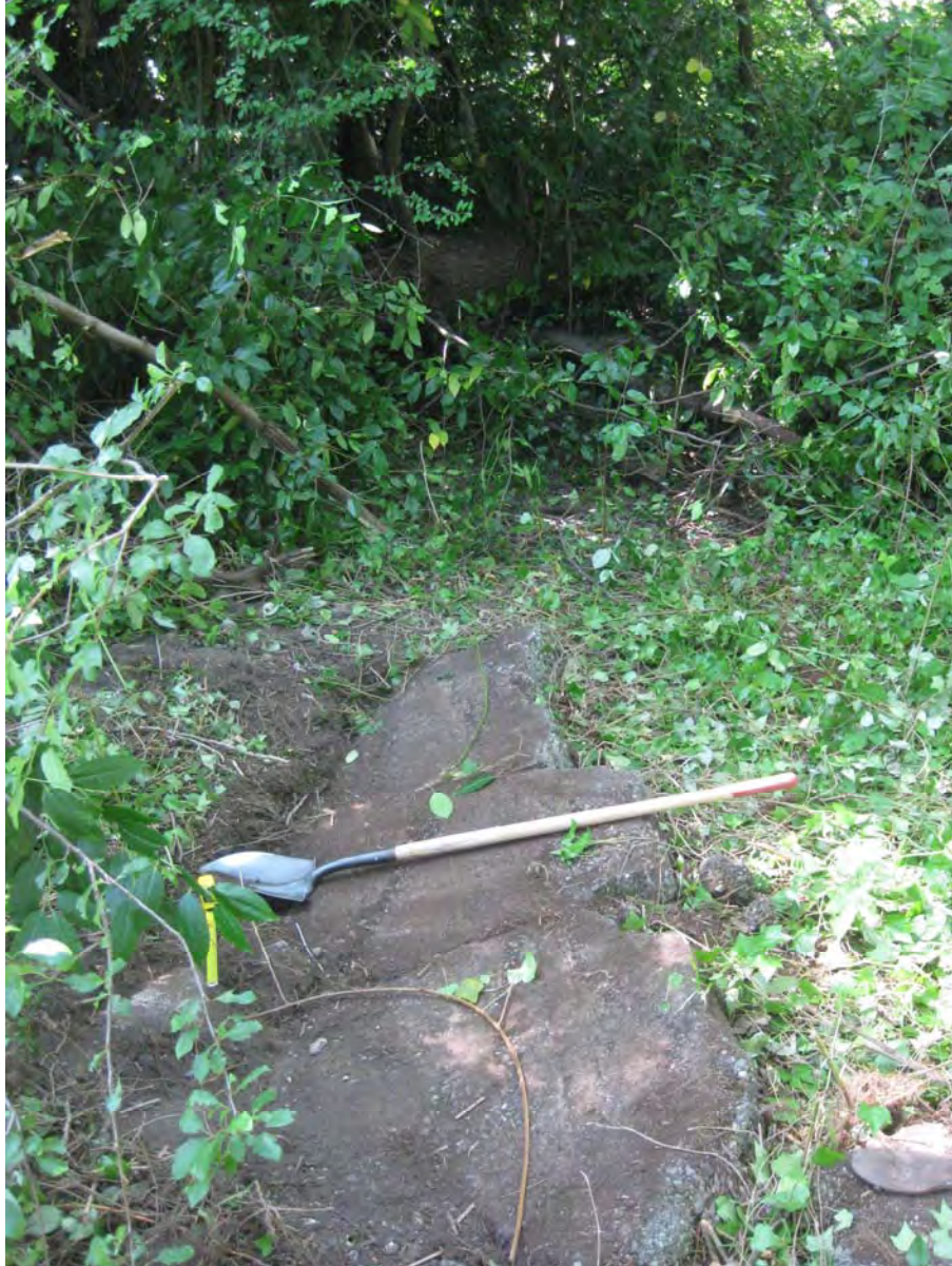
Figure 5. Remnant of concrete walls in dense vegetation, view south.
