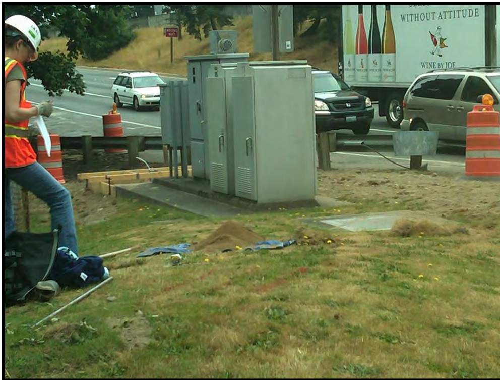
Figure 2-10. Jenny Dellert at Shovel Probe 12-1 and utilities in Area 12, view south
