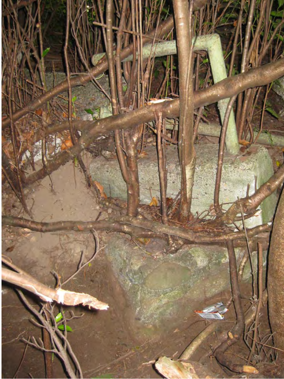
Figure 6. Remnant of concrete steps, handrail, and intersecting rock wall in dense vegetation, view west.
