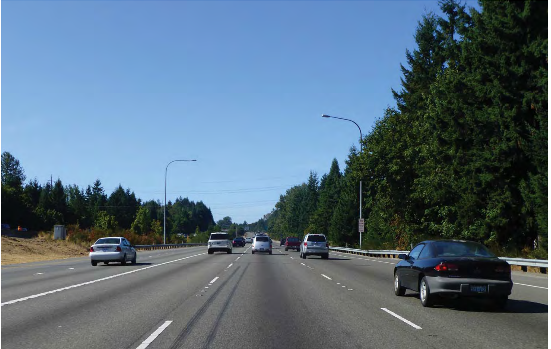
Figure G-130. Viewpoint 41 I-5 Southbound at 50th Avenue West View to the south Existing View
