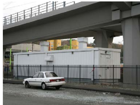
Example of a Traction Power Substation
