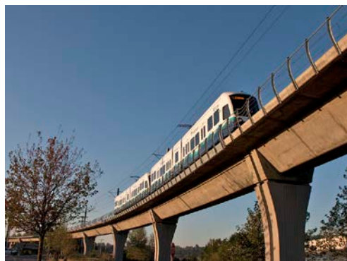
Light Rail Train with Overhead Catenary Wires in Tukwila, WA
