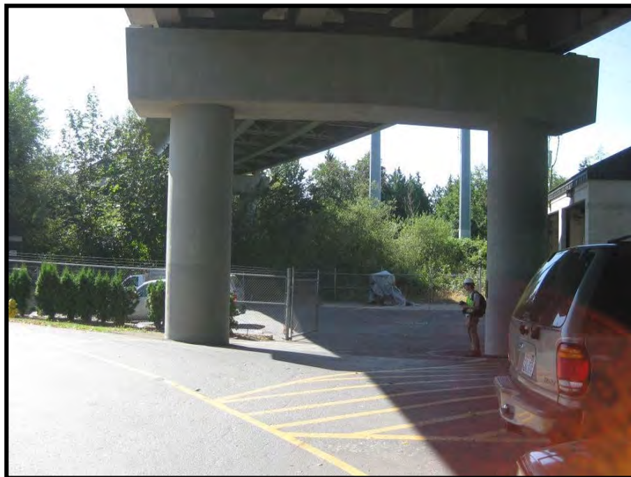
Figure 2-7 View of paved and fenced City of Lynnwood Pump Station No. 10 (Parcel 170 adjacent to park-and-ride), view south
