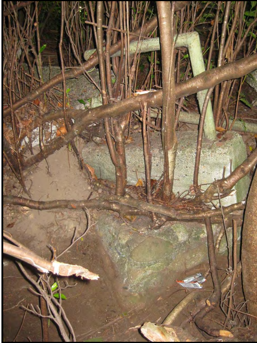
Figure 3-5 Overview of concrete steps, handrail, and intersecting rock wall, view west
