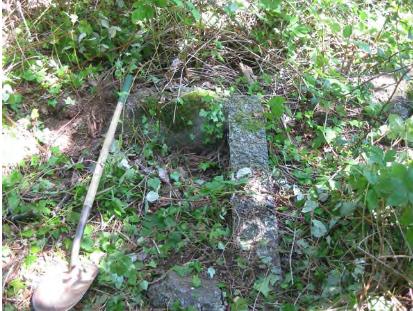
Figure 4. Remnant of concrete walls in dense vegetation, view north.
