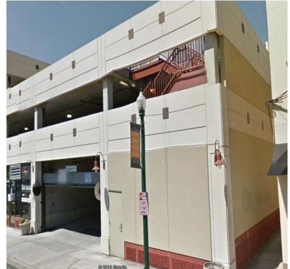
2 ½ story view of Puyallup's DSHS garage (3 levels of parking)
