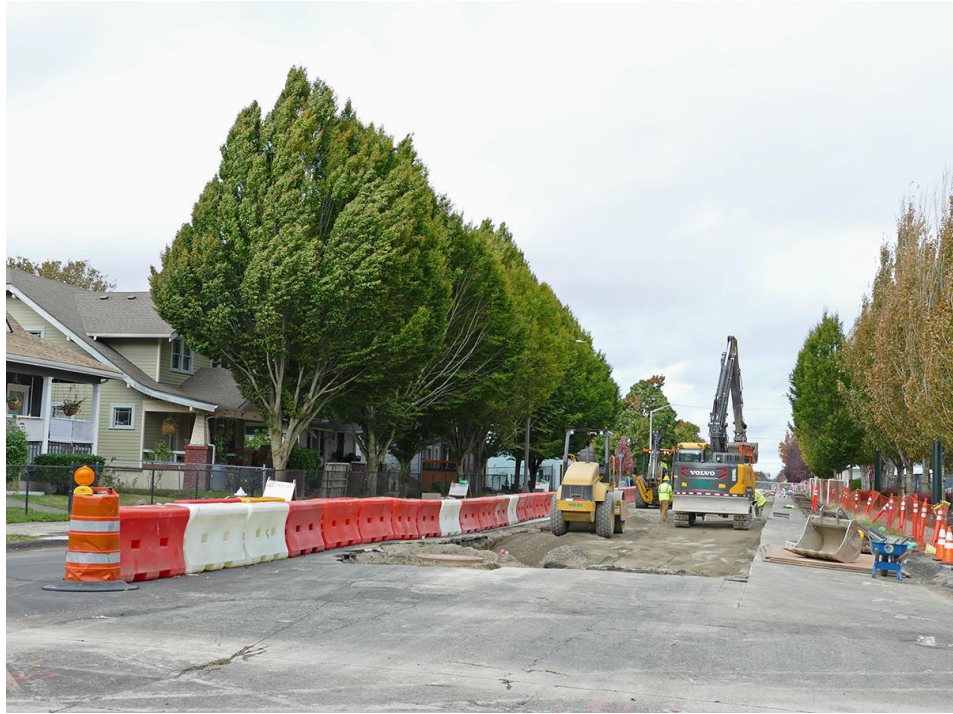
Excavation for track slab at S. 18 th
