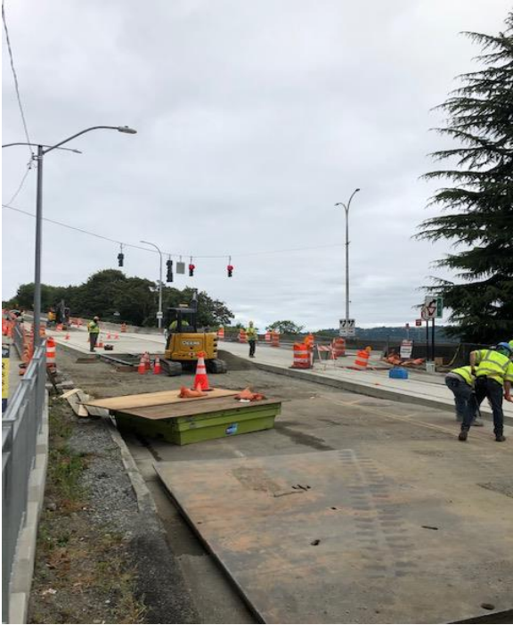
Stadium Way/I-705 track work in progress
