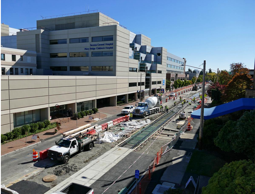
Track installation at Tacoma General
