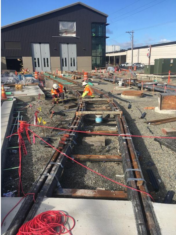
Special track work in progress at yard
