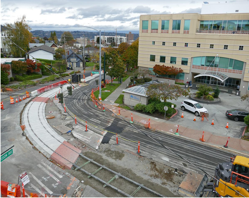
Work in progress at Division Ave. and MLK
