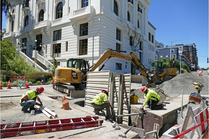
Utility work on Commerce St.
