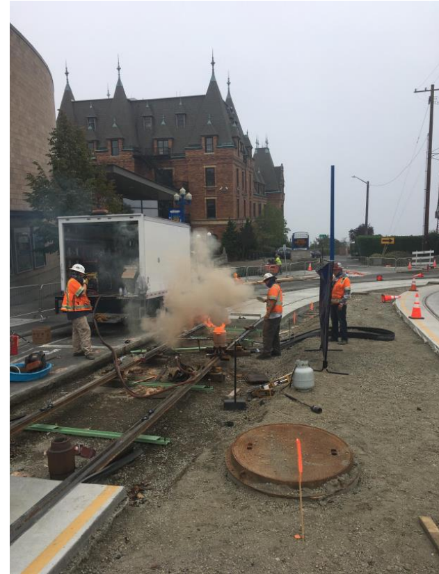
Welding outbound rail at curve
