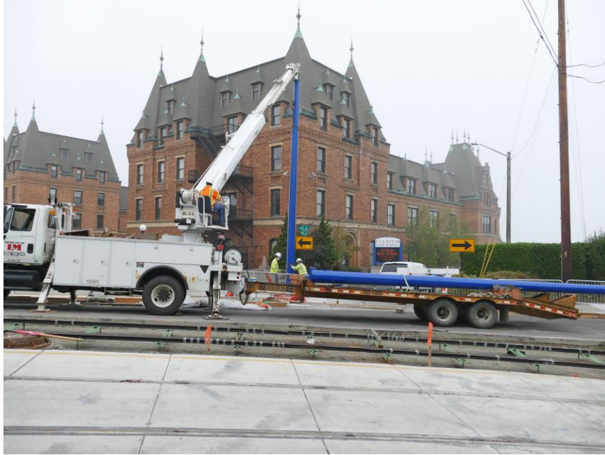
OCS Pole installation at Stadium High School
