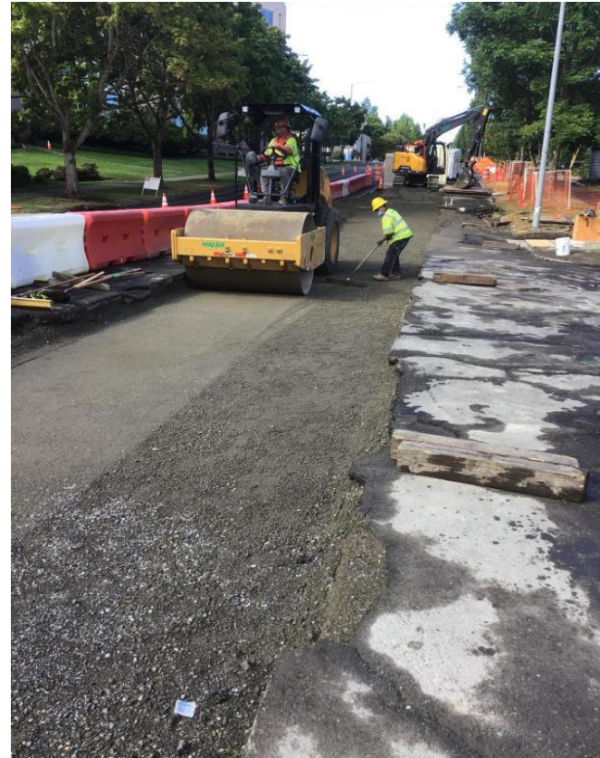
Grading for outbound track slab on Division Ave.
