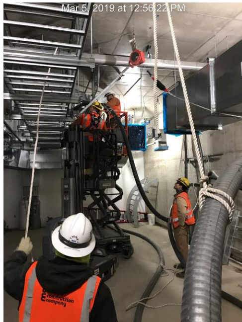
Power Cable Installation at UDS
