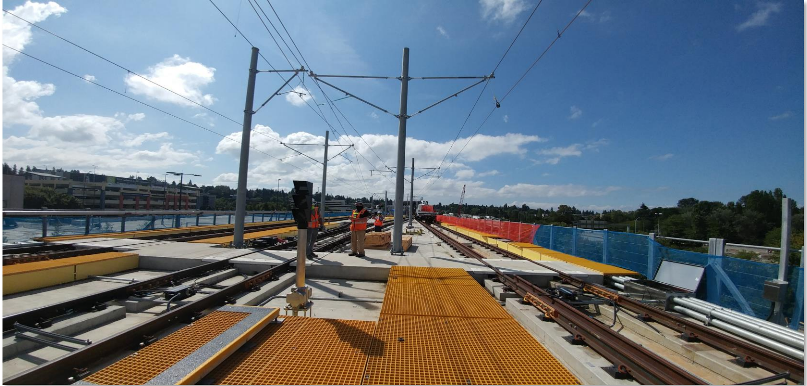
Looking North from Northgate Station at Overhead Catenary System (OCS)
