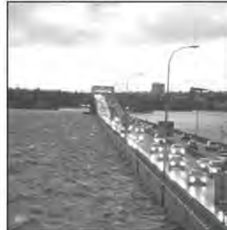
Strong waves batter the SR 520 floating bridge during a windstorm
