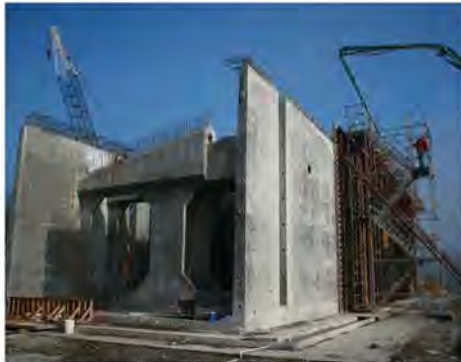
Crews built a test pontoon at Satsop Business Park. The test pontoon was approximately one-sixth the size of a proposed SR 520 bridge pontoon.
