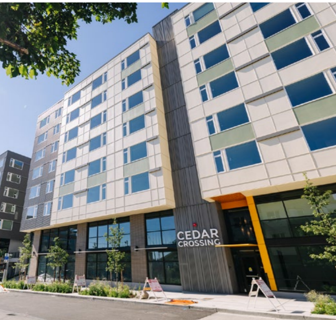
Meeting a critical regional demand: Adding new affordable housing in Seattle.
