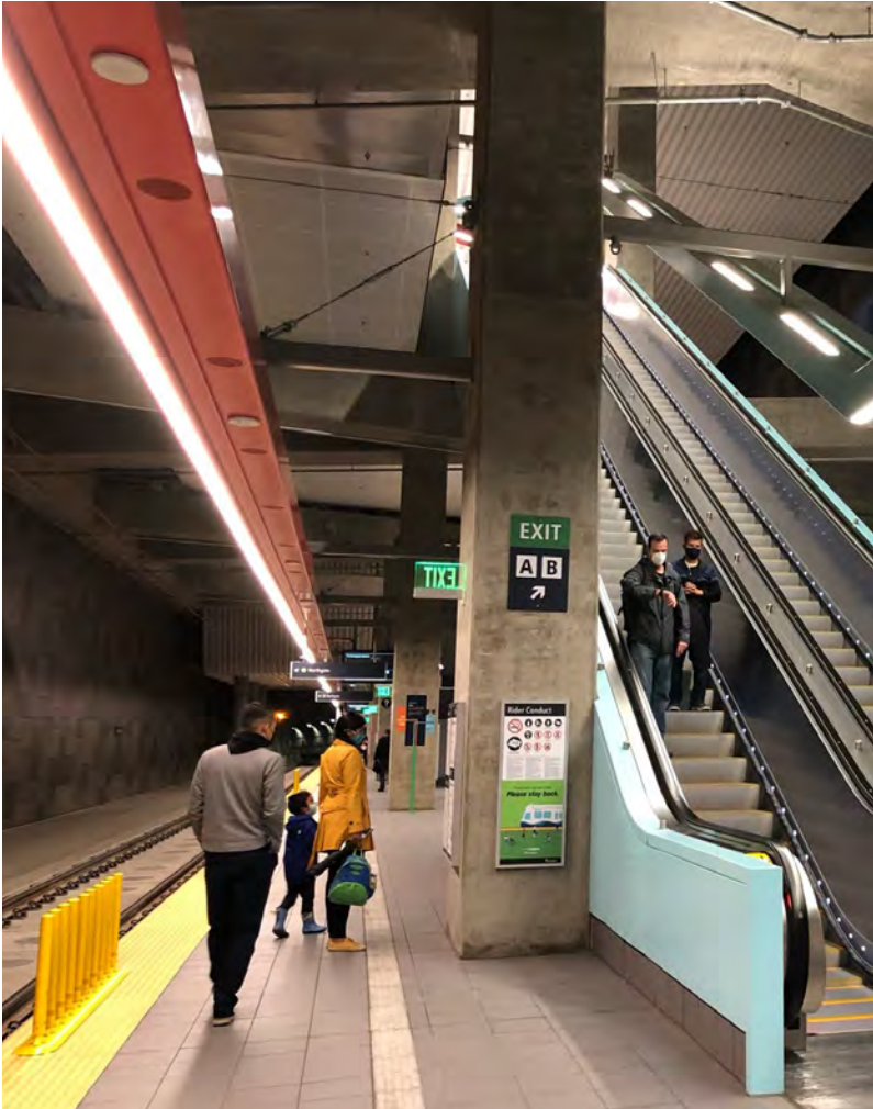
Figure i for 3.3.3 - An example of a maintenance-accessible Formed Metal Enclosure (FME) used to house lighting, speakers, and attach signage while concealing conduit and cables..
