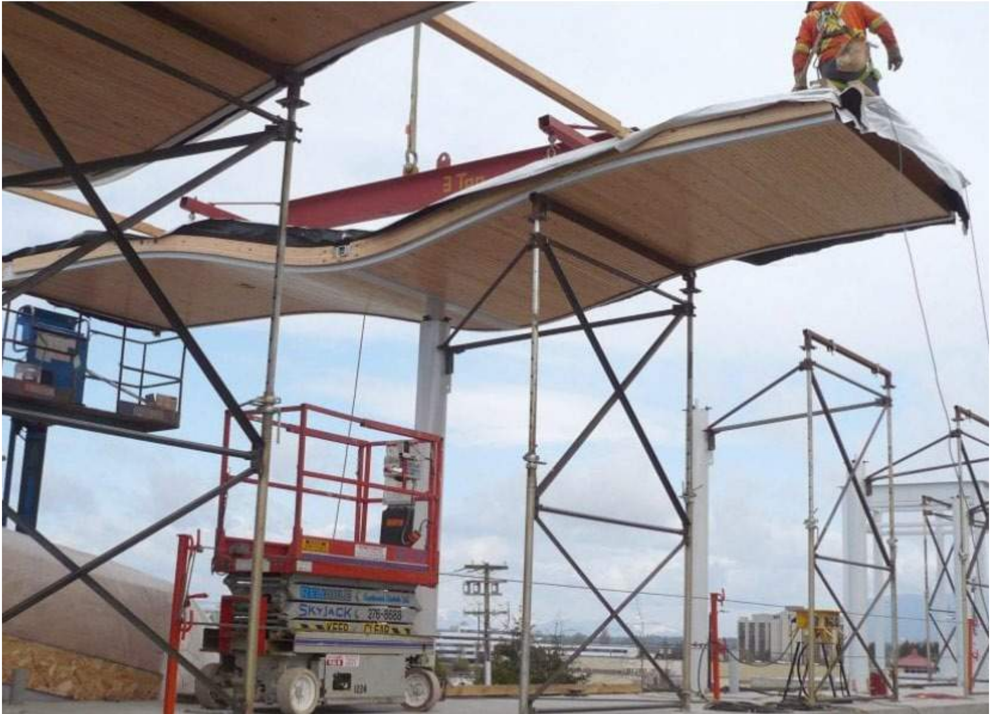
Figure i Hoisting prefabricated elements into place
