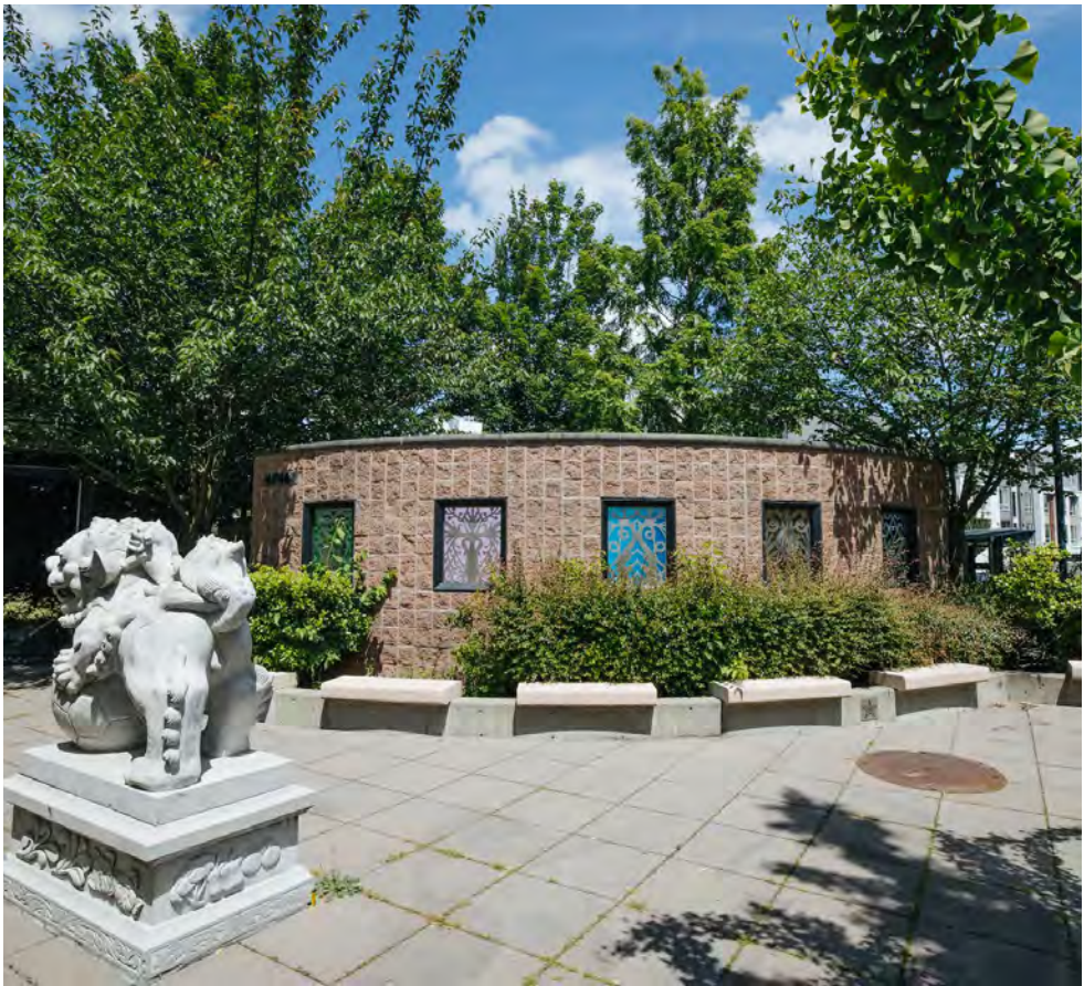
Figure iii for 3.3.12 - TPSS screened from view with concrete masonry and landscaping
