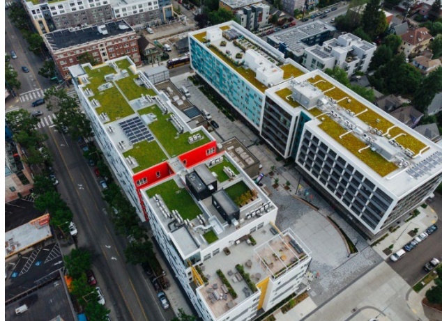
LEED Certified: The Capitol Hill Station buildings feature green roofs and photo voltaic panels, two energy efficient features that helped the projects achieve LEED Platinum.
