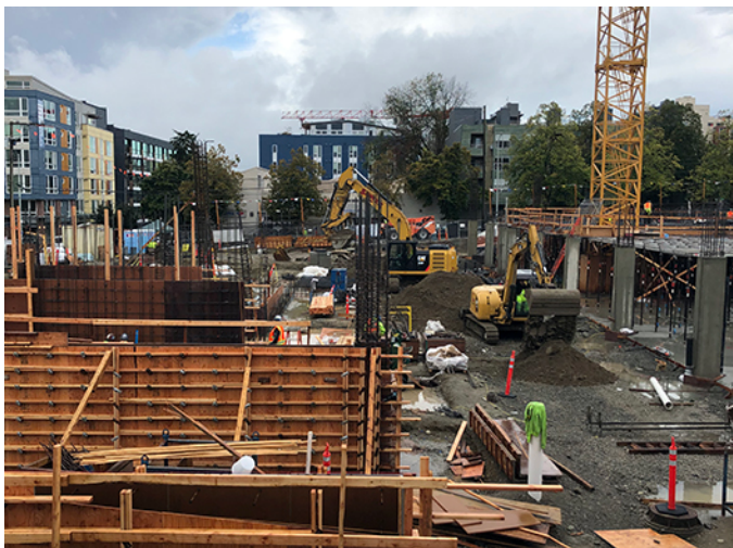
Concrete work at the Cedar Crossing project in Roosevelt continued in Q3 2020. Due to the project's close proximity to the underground station, Sound Transit and the developer have a construction coordination plan that addresses safety, settlement monitoring, haul routes, etc.
