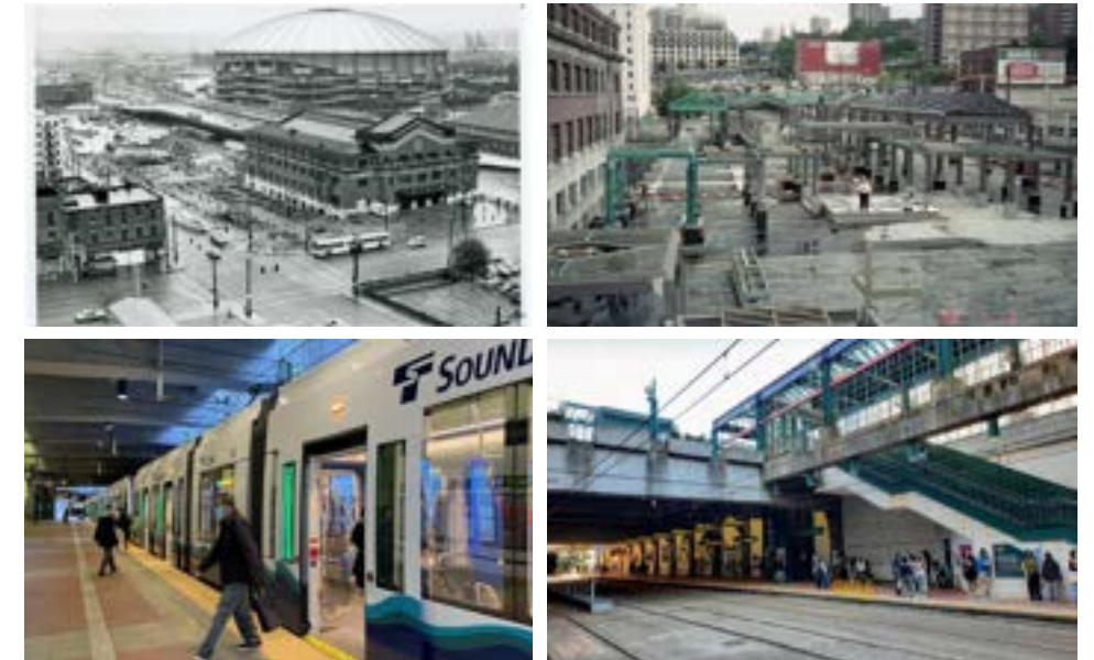
Figure 1.05. Downtown Tunnel. Top: Two photos showing the construction phase of Chinatown-International District Station plaza and tunnel. Bottom: Two photos of the transit tunnel in use in recent times. Sources: Seattle Municipal Archive; Sound Transit.
