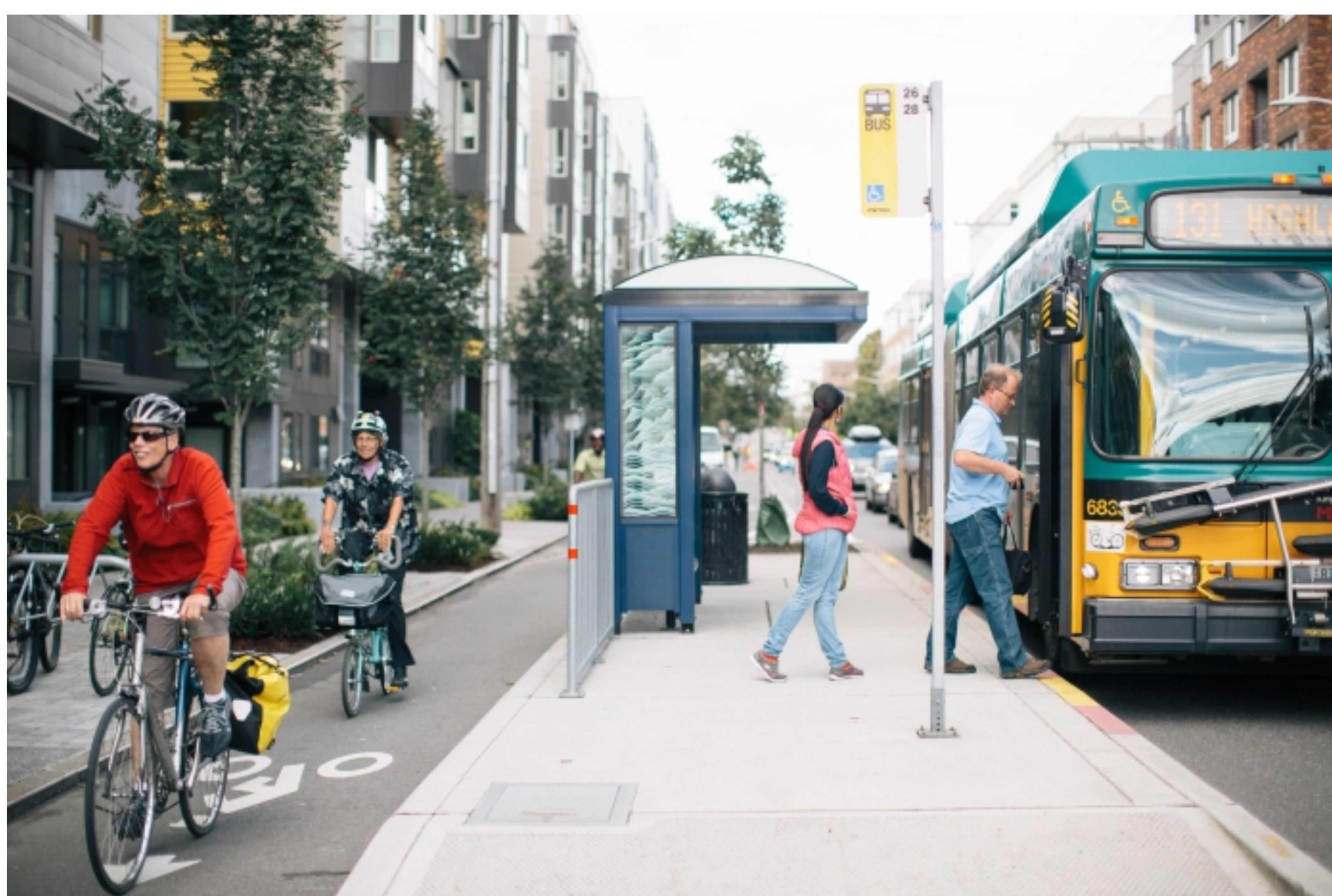
Example of a floating bus stop in Seattle (source: pedbikeimages.org / Adam Coppola Photography).
