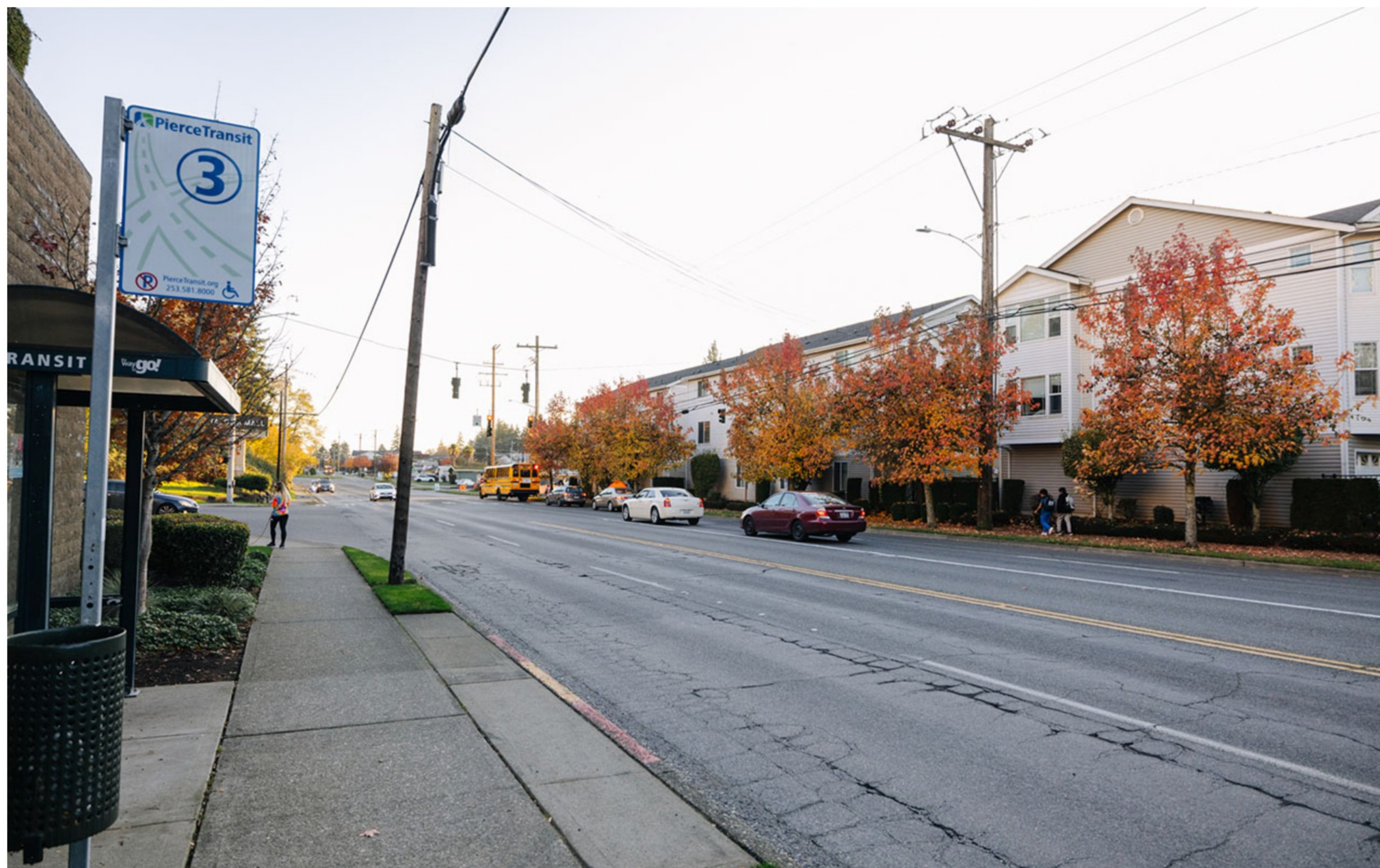
Current view of a Pierce Transit bus stop on South Pine Street, looking south toward the intersection with South 45th Street. The current roadway has two travel lanes in each direction.
