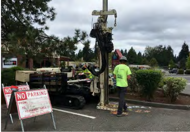
Figure 7-12 Extraction of core LFP-1 on the upper landform within the proposed Lake Forest Park Park-and-Ride garage location, view north
