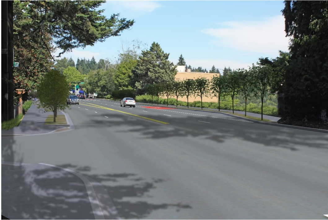
Figure 3: VP 08 — SR 523 (NE 145th Street) Looking East near 12th Avenue NE, with Project in Place
