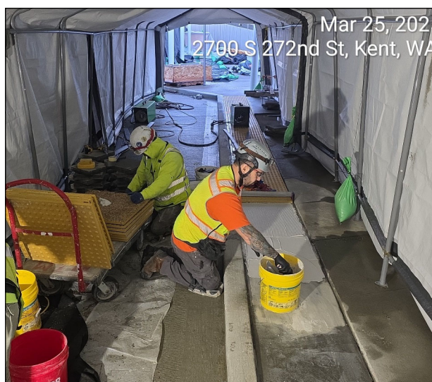
Star Lake Station Bus Loop Paving Tile Installation
