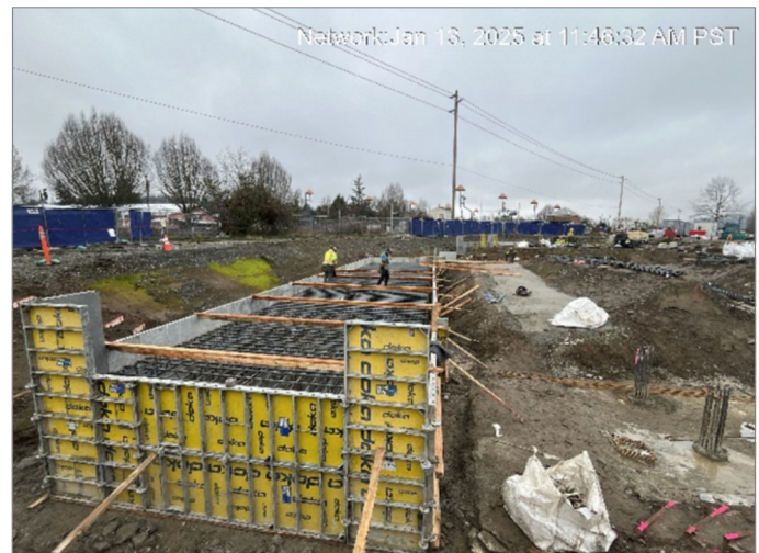
Forming & pacing pile caps/grade beams at Sumner
