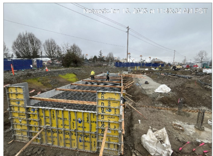
Forming & pacing pile caps/grade beams at Sumner
