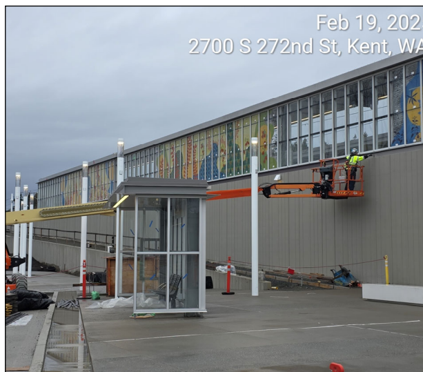
Star Lake Station West Wall C– Channel HPC Apply
