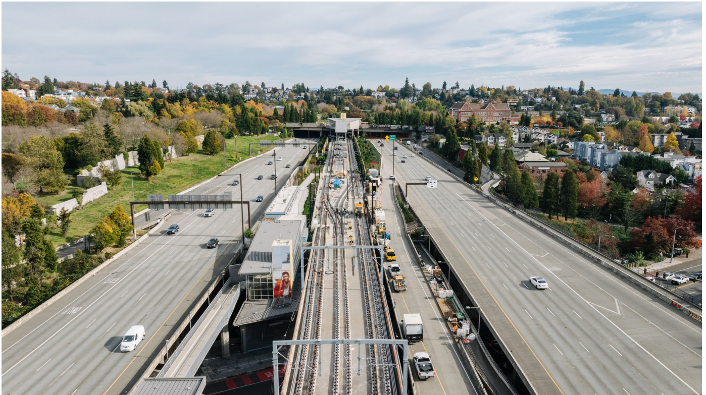
Aerial view of Judkins Park Station and Guideway
