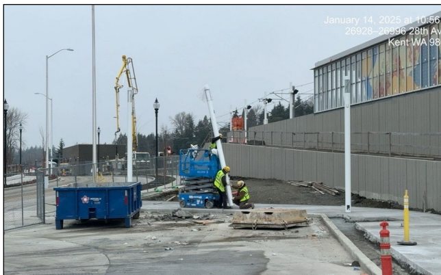
Star Lake Station Plaza Light Pole Placement
