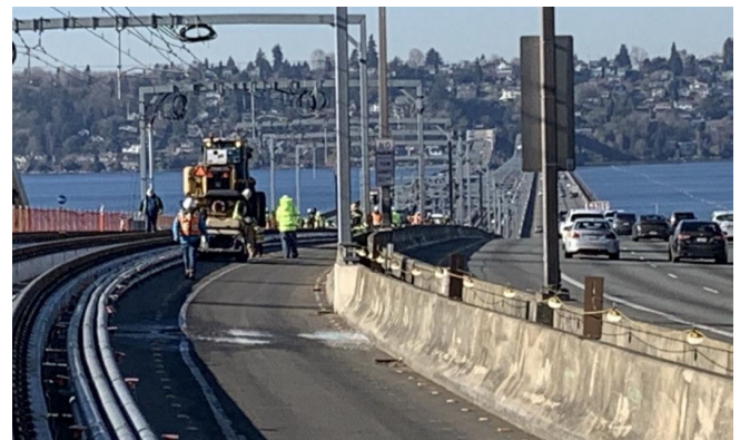
I-90 Signals Installations
