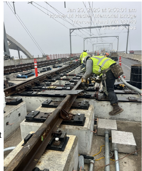
E130: Installing shimming and other track materials on floating bridge westbound
