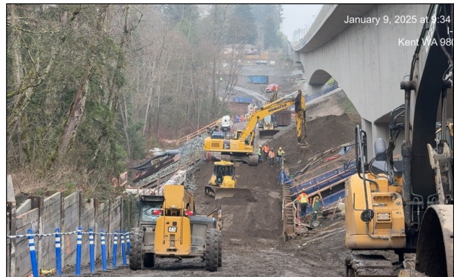
Structure C Wall Backfill
