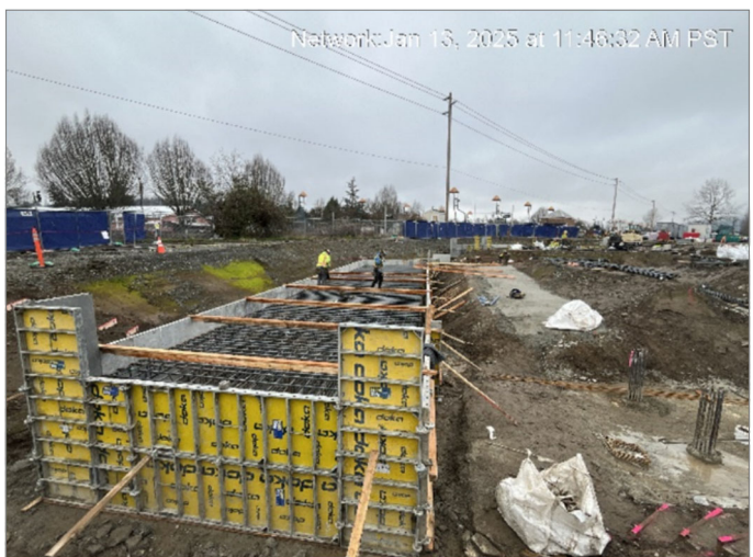
Forming & pacing pile caps/grade beams at Sumner
