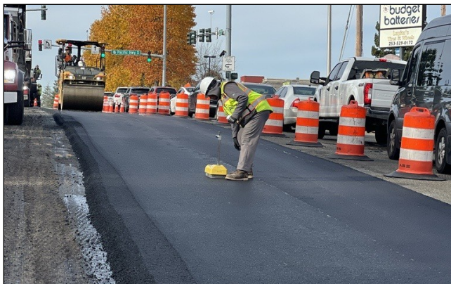
F210– Site 5 Compaction Test at 272nd ST Paving
