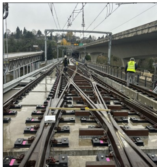
Punchlist check of rail geometry and shim installation, west approach double crossover
