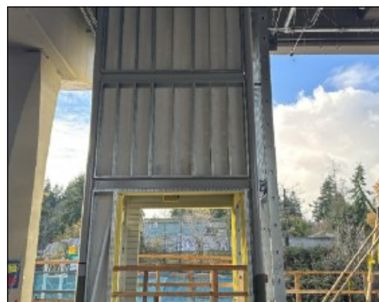
Elevator framing
