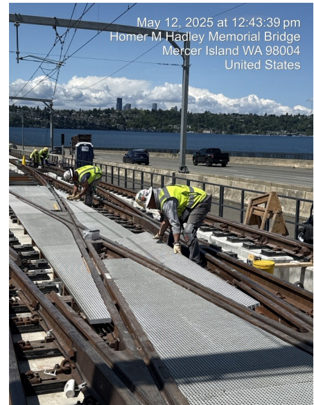
E130: Crew is performing dry fitting of fiberglass grating at crossover
