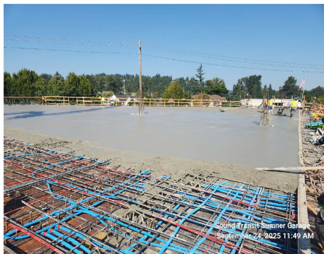
Sumner: Northwest at the Level 2 Zone 4 elevated deck concrete pour.
