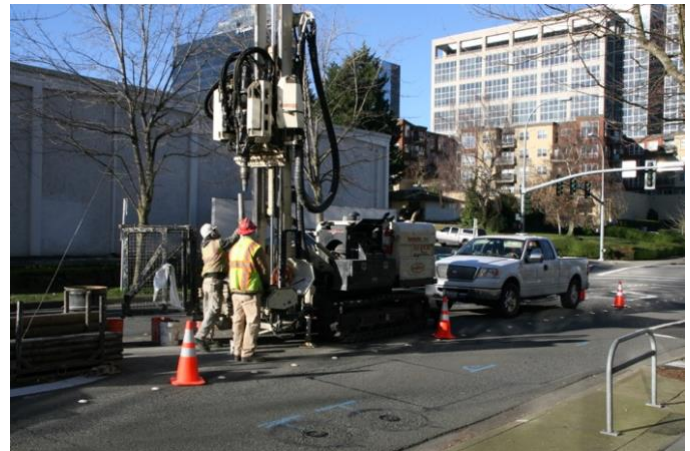
Example of geotechnical drilling equipment
