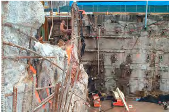
STEP 4: DEMO PORTION OF SLURRY WALL BELOW KEXP
