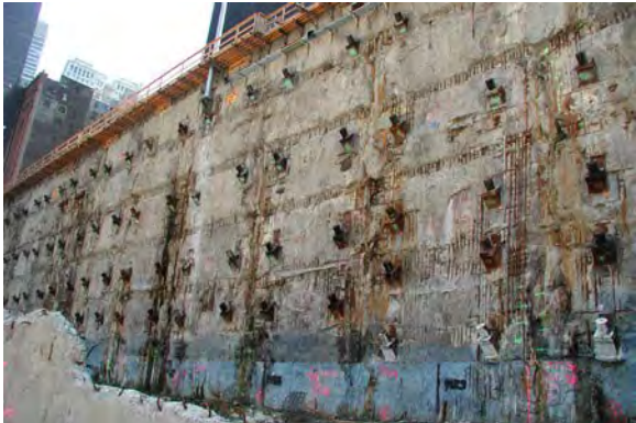
STEP 3: BUILD SLURRY WALL
