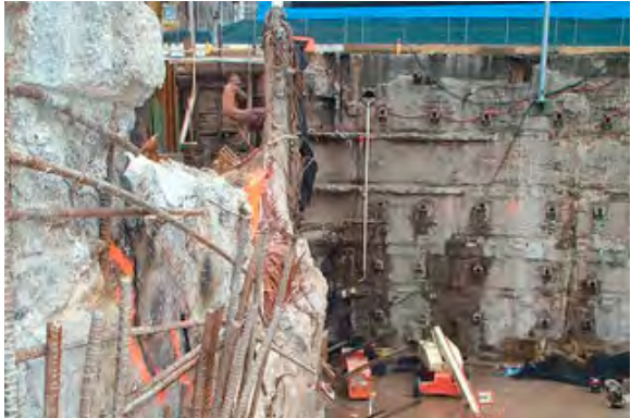
PHASE 4: DEMO PORTION OF SLURRY WALL BELOW KEXP
