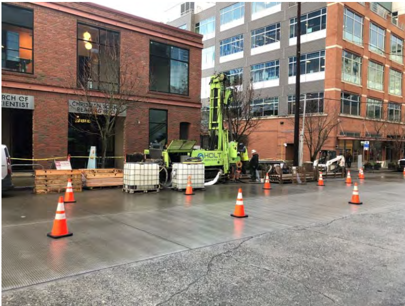
Geotechnical drilling rig in South Lake Union
