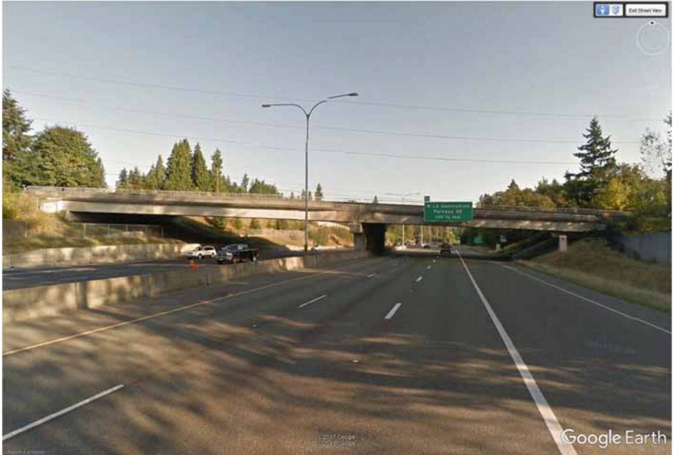
Exhibit D-5. Northbound View from SR 520 of the NE 60th Overpass (Approximately 200 Feet Away)
