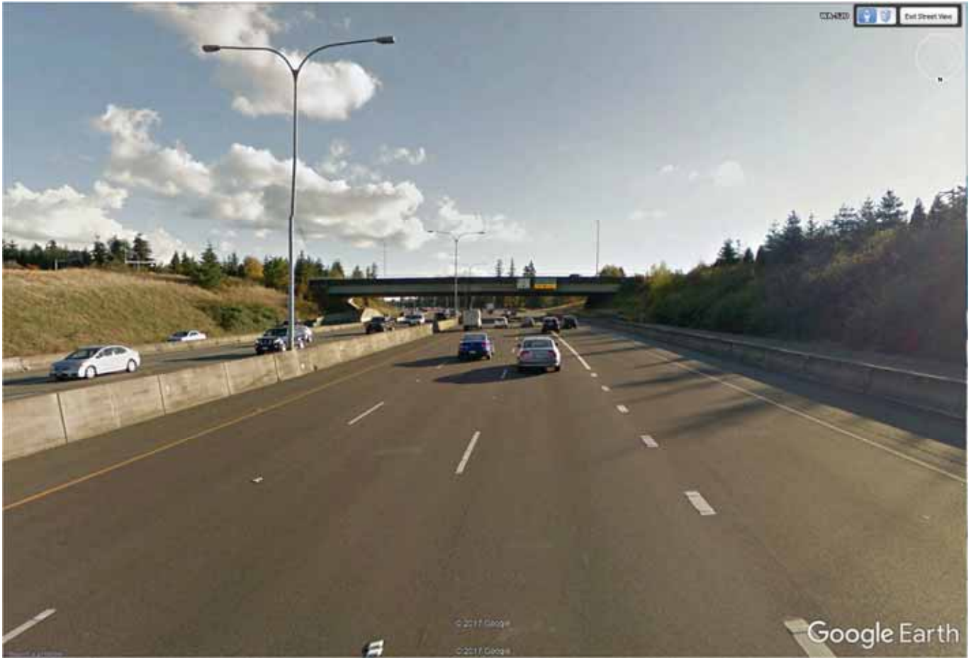
Exhibit D-7. Southbound View from SR 520 of the NE 51st Street Overpass (Approximately 400 Feet Away)
