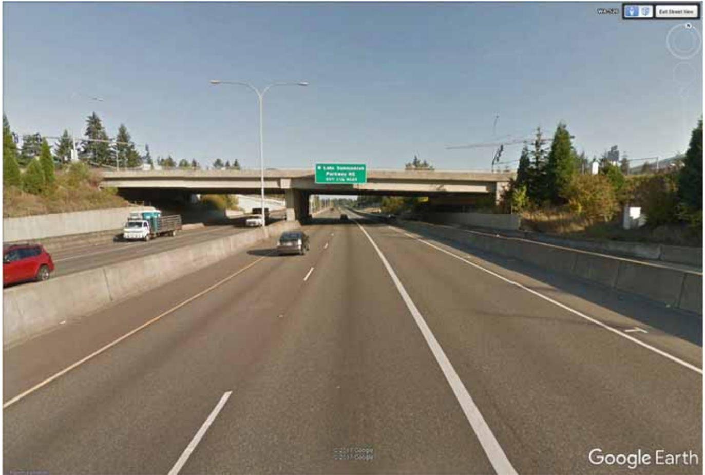
Exhibit D-3. Northbound View from SR 520 of the NE 40th Street Overpass (Approximately 200 Feet Away)
