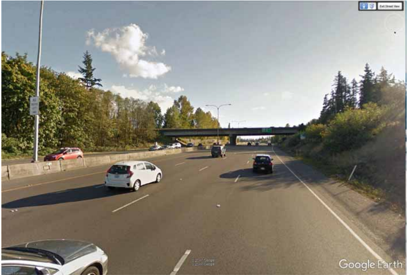
Exhibit D-6. Southbound View from SR 520 of the NE 60th Overpass (Approximately 400 Feet Away)
