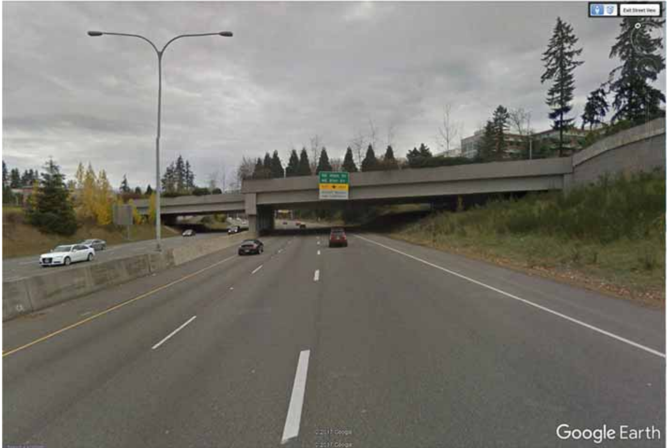
Exhibit D-2. Northbound View from SR 520 of the NE 36th Street Overpass (Approximately 200 Feet Away)
