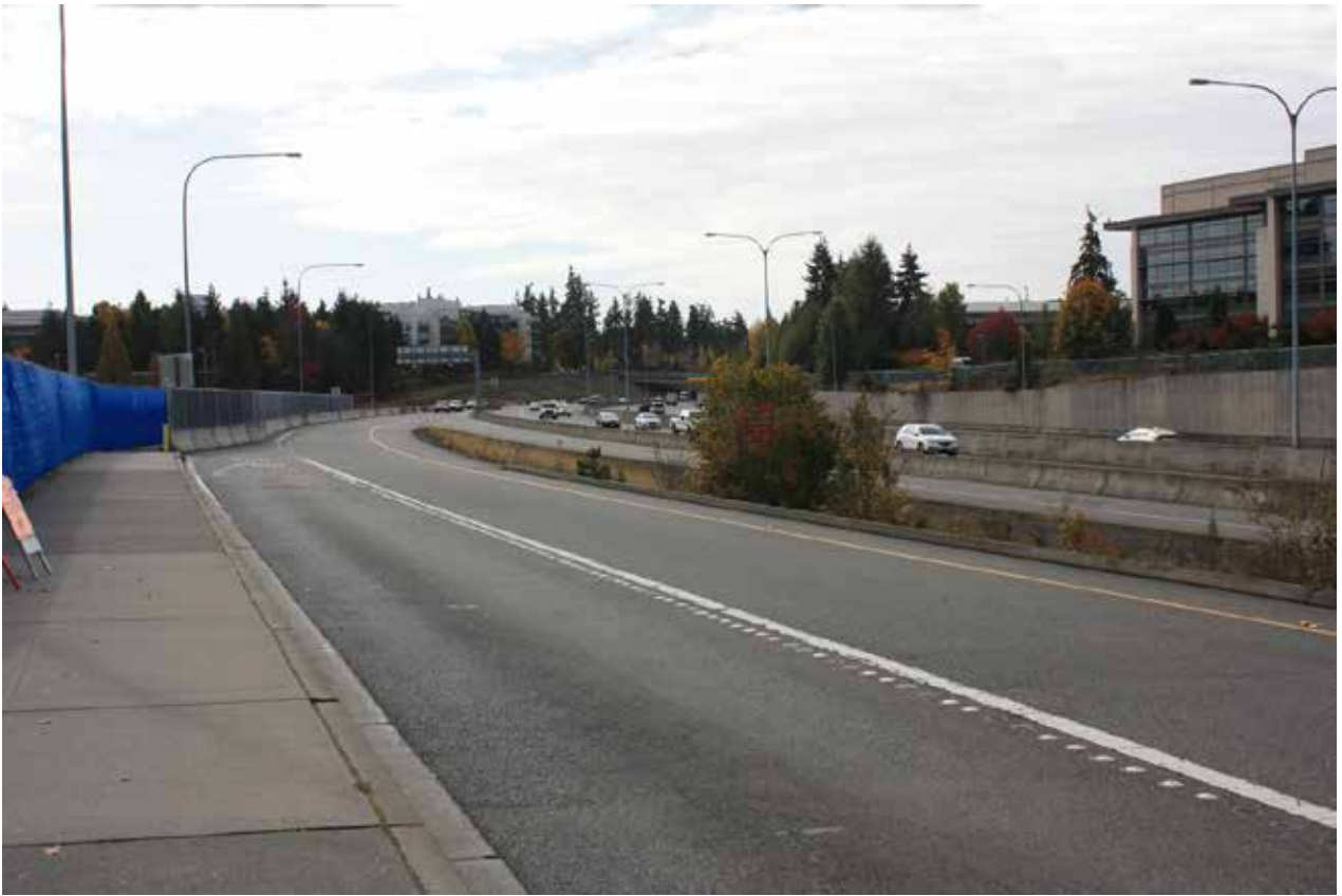
Exhibit 3-2a. Existing Conditions from East Side of SR 520 (Looking South)
