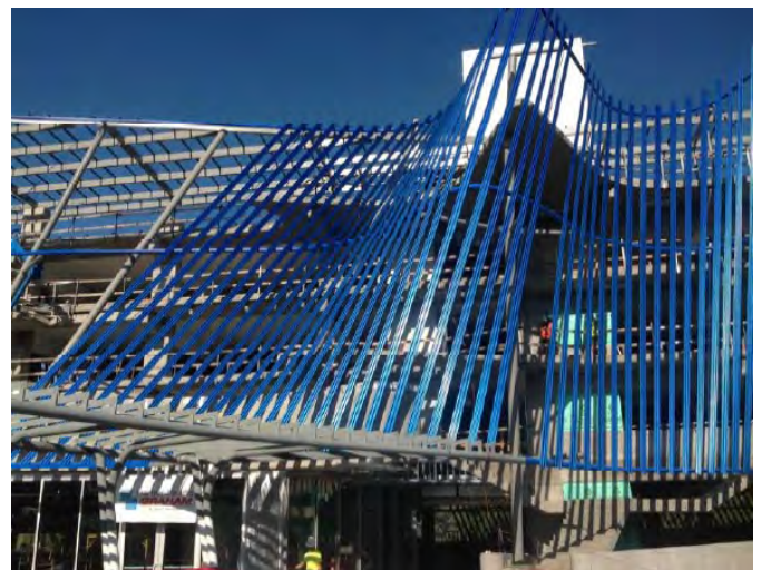
Façade installation ongoing at the garage.
