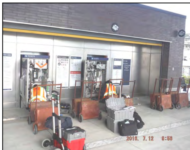
TVM installation at the Angle Lake Station.
