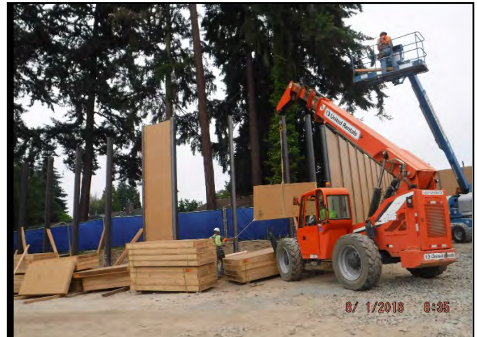
South Portal looking NW –installation of sound wall parcels.
