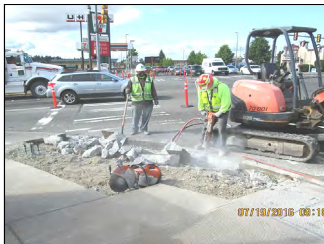
Demolition of curbs and gutter at S. 200th St. corner.
