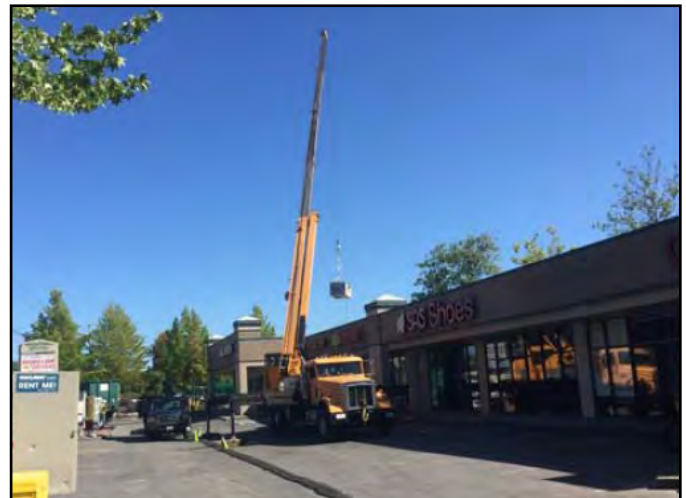
Removing rooftop A/C.
