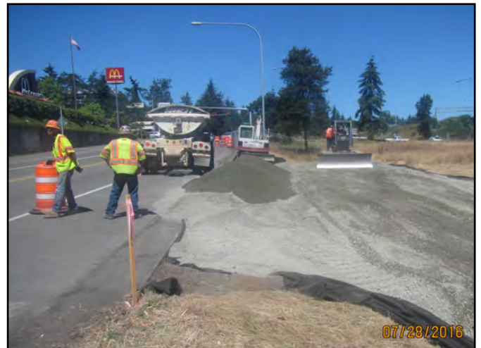
Delivering gravel at Pole site 4.
