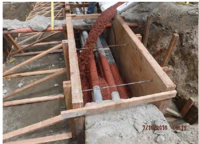
E330 FTB placed in Trench 2 PSE duct bank
