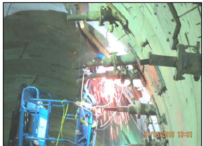
Welding freeze pipe collar in SB tunnel at CP34.
