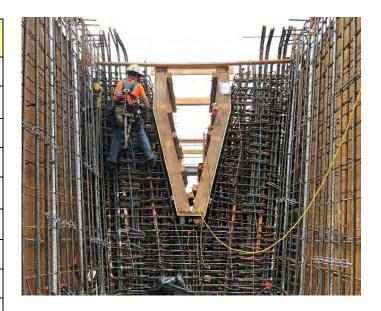
Tying rebar on wall formwork on the pier table along I-90 Flyover support structure.
