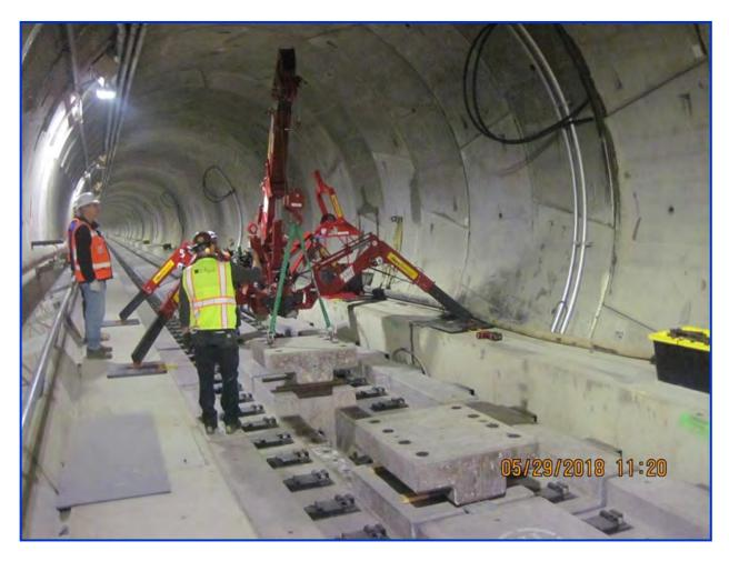
N830 (Mass Electric) hoisting floating slab trench cap for EMI cable work Northgate Link Extension
