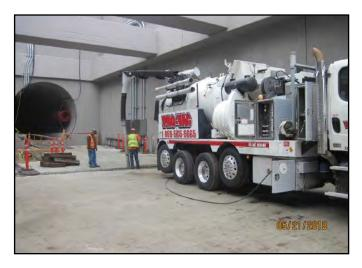
Crews removing the backfill materials from the N125 concrete cast drainage trench at MLP prior to the start of construction on the MLP stair tower.
