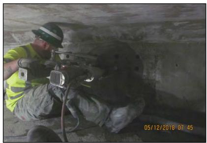
E130 Seattle to South Bellevue: Core drilling in very confined space in the bridgespan on I-90
