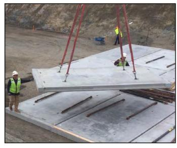
Placing prefabricated concrete panels during installation of the underground infiltration vault.
