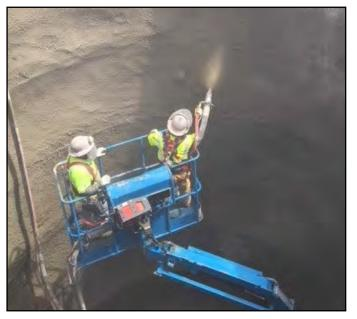
Applying 1.5" smoothing layer at mid-tunnel shaft
