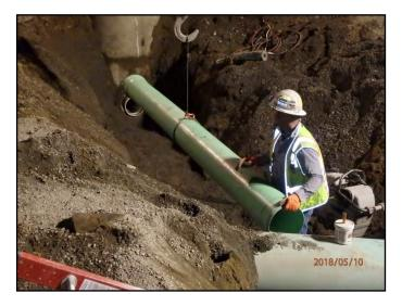
Installation of the drainage pipe and drainage structure on 130th Ave NE facing west.
