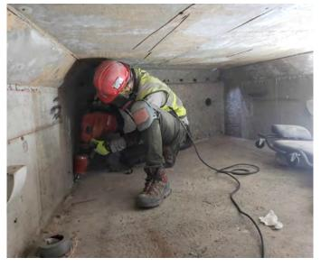
Concrete surface preparation work in a pier underneath I-90 in the Judkins Park Station site.
