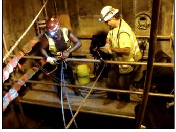
Installing tendons for post tensioning inside floating bridge pontoon.
