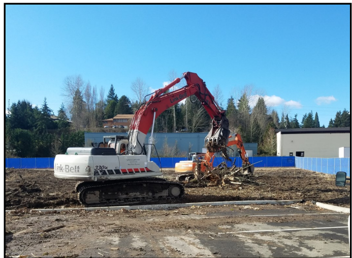
Clearing and grubbing at the site.
