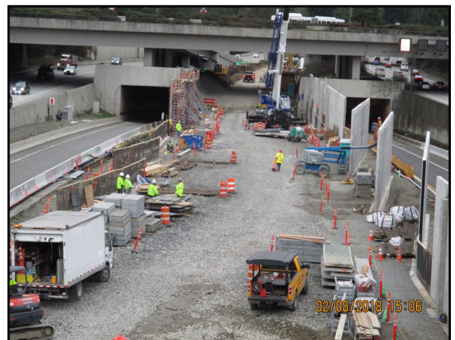
Sound Wall erection at the Mercer Island Station site.
