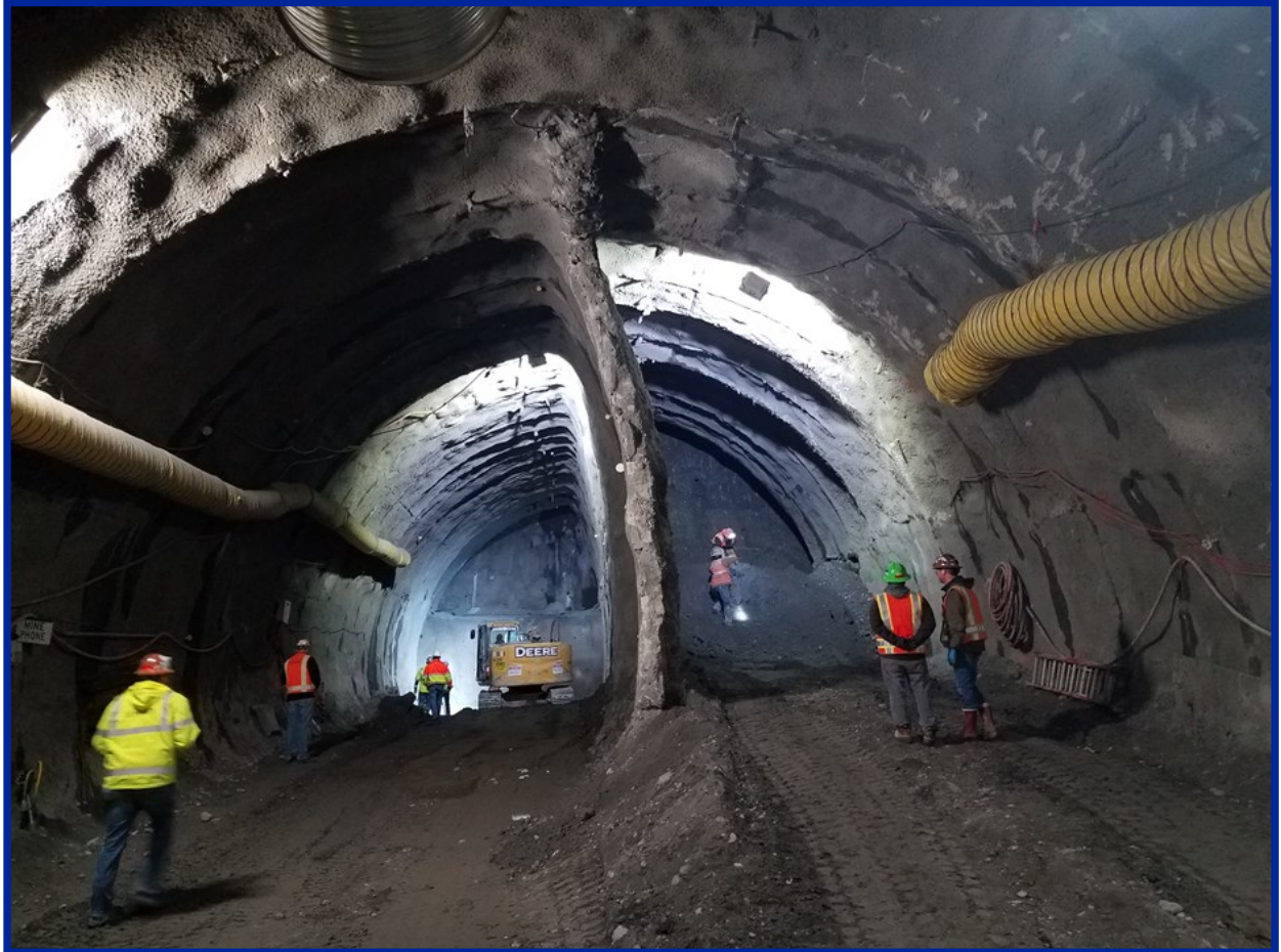
Downtown Bellevue Tunnel– Excavation of Enlarged Tunnel Section (East Link Extension)
