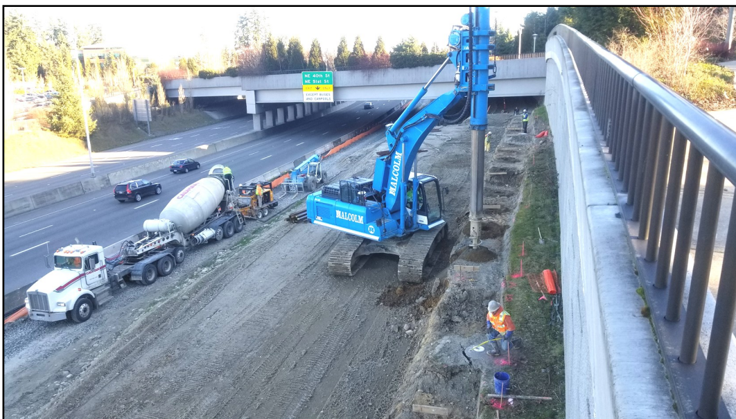
E360 SR520 to RTC- Installation of vertical elements wall
