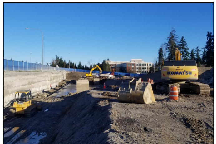
Wall S8 –Soil Nails and WSDOT Vault Demolition along SR-520
