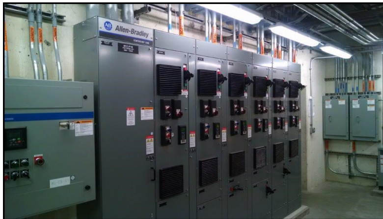
Jet fan MCC electrical controls, Mt. Baker Ridge Tunnel
