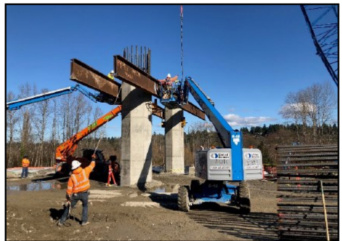
Setting false work for the station platform.
