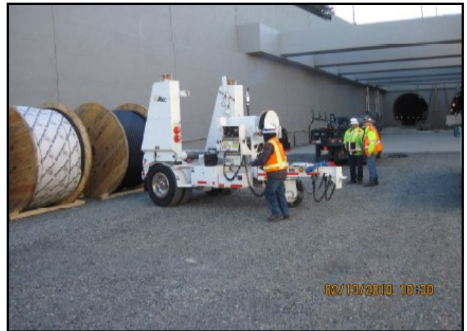
Liberty Electric loading a spool of 26kV with the Altec cable handler, at the MLP site, and transporting it into the tunnel to be installed.
