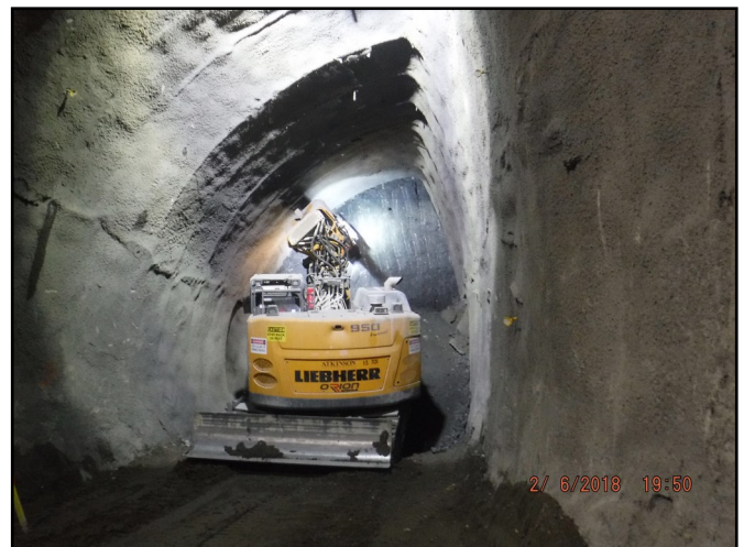
Excavating tunnel top heading.
