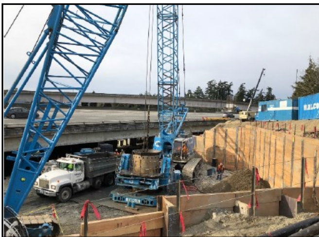
Installing drill shaft at I-90 Flyover.
