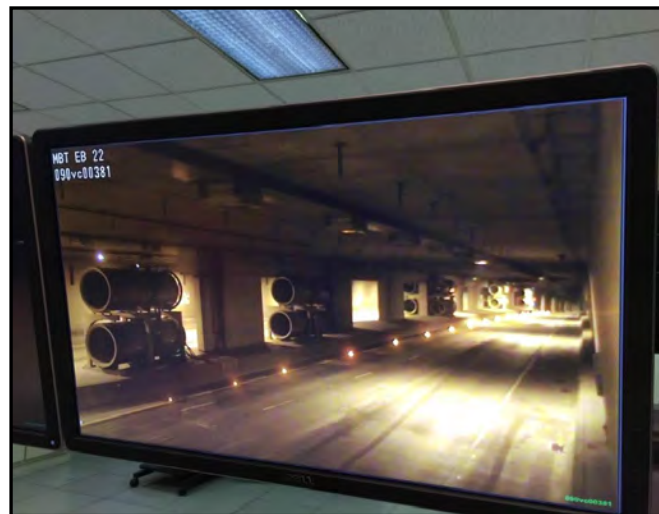
CCTV image of in-pavement lighting & jet fans
