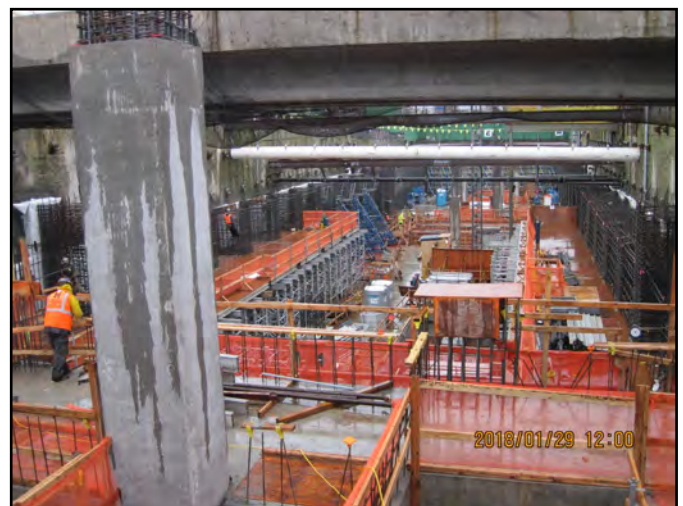
RVS view of station box activities looking south.
