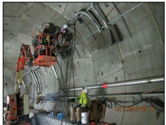
NB Tunnel: Elcon wire pulling from CP38 towards RVS.
