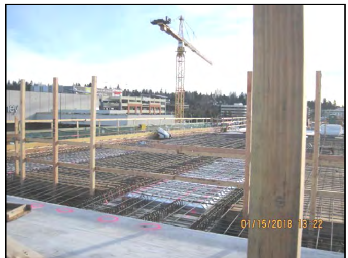
Span B4 rebar installation—looking south.
