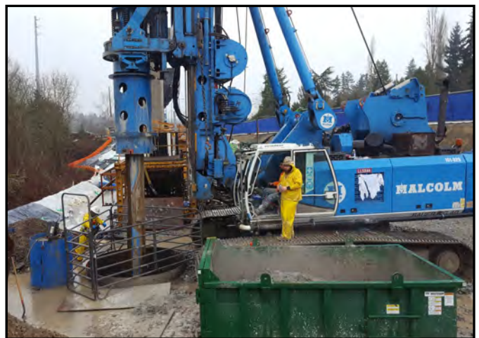
Shaft coring along I-90 and Bellevue Way.
