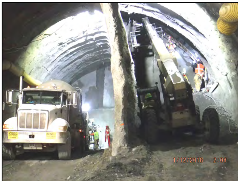
E330 Tunnel excavation- Lattice girder installation at top heading
