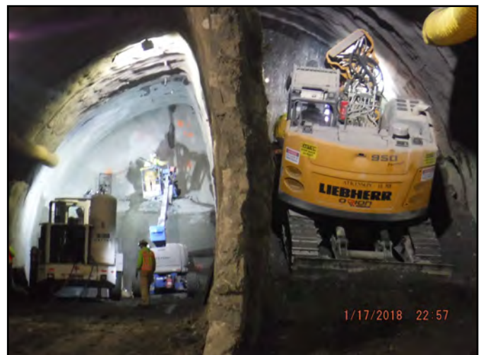
6-Heading SEM Excavation Continues.
