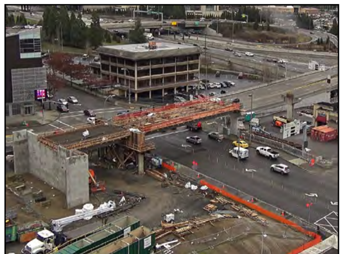
Span 1 and 2- Aerial Guideway over 112th Ave NE Bellevue (Area 4)
