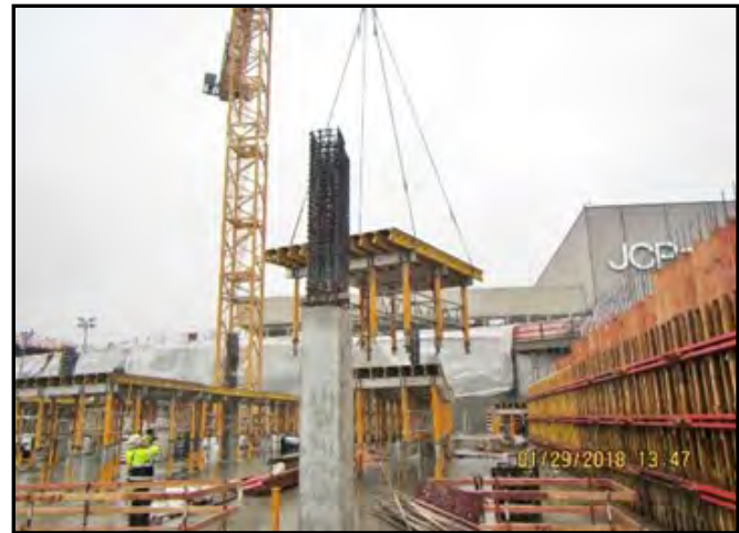
Ongoing work at Northgate Station setting Peri falsework.
