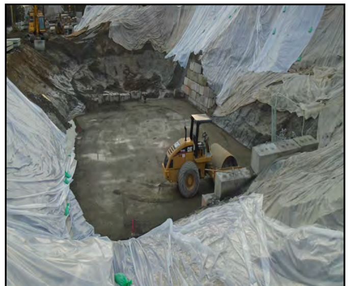
Vault excavation at the corner of 136th Place and Spring Boulevard
