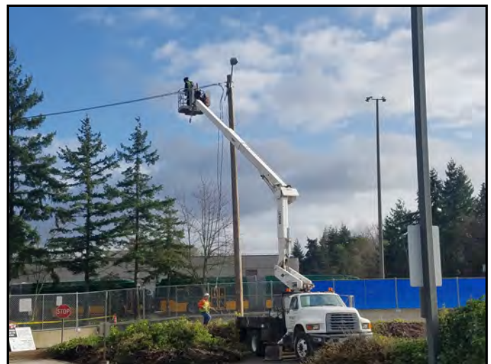
Working on temporary overhead powerline.
