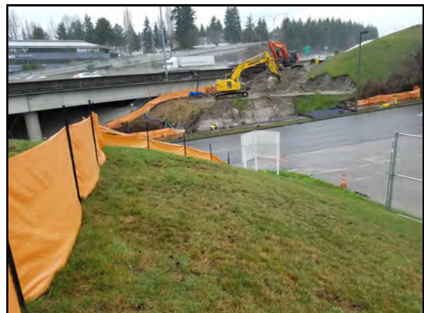
Excavation of shaft construction pad along SR-520
