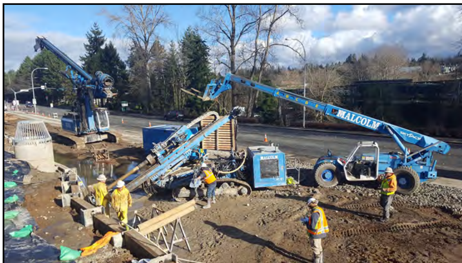
E320 South Bellevue- Installation of soldier pile tie backs SE 6 th St and 112 th SE
