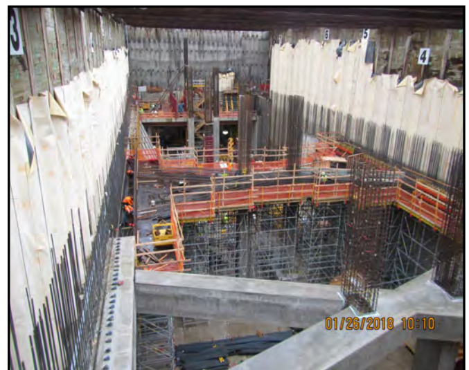
U District Station – Overall station looking north.
