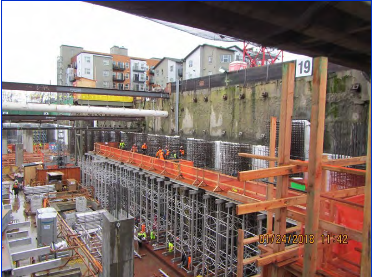
Installation of formwork and rebar for the walls and elevated slabs at the Roosevelt Station (Northgate Link Extension)
