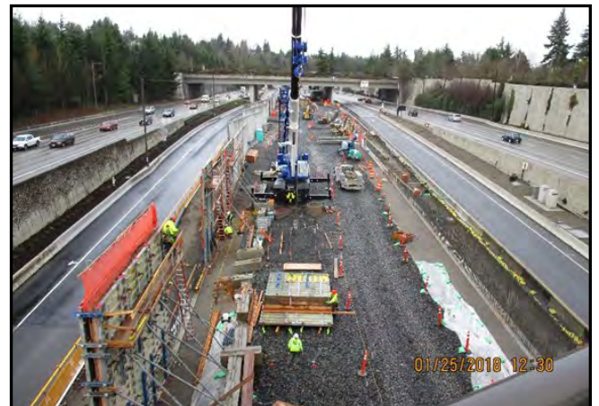
Sound Wall installation at the Mercer Island Station site.
