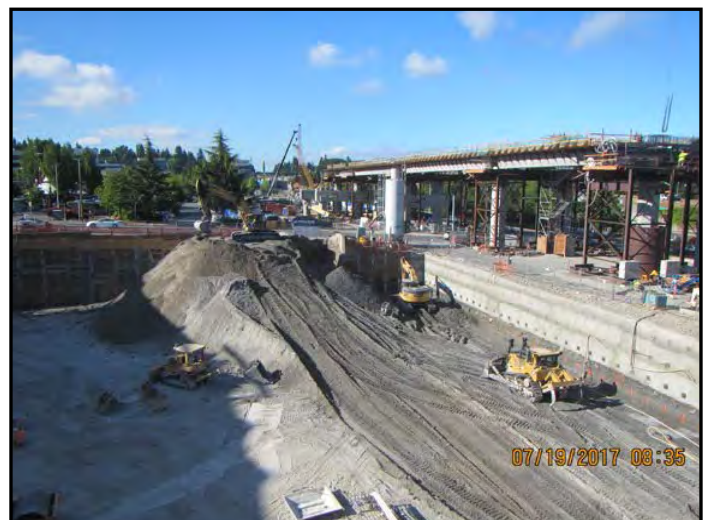
Garage mass excavation looking south.
