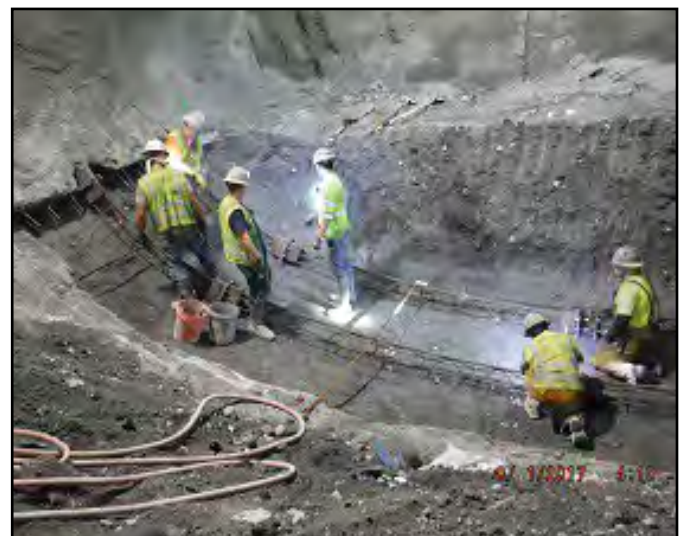
Installing lattice girder at invert.
