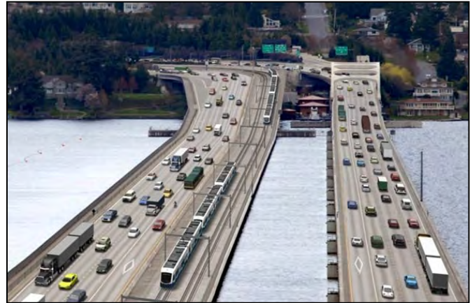
The project, when completed, will enable 24/7 HOV access on I-90 between Seattle, Mercer Island and Bellevue.
