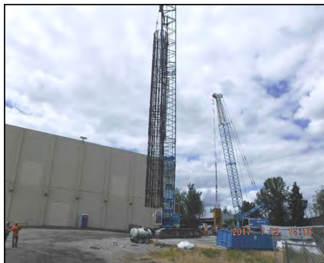
Workers continued drilling shafts.
