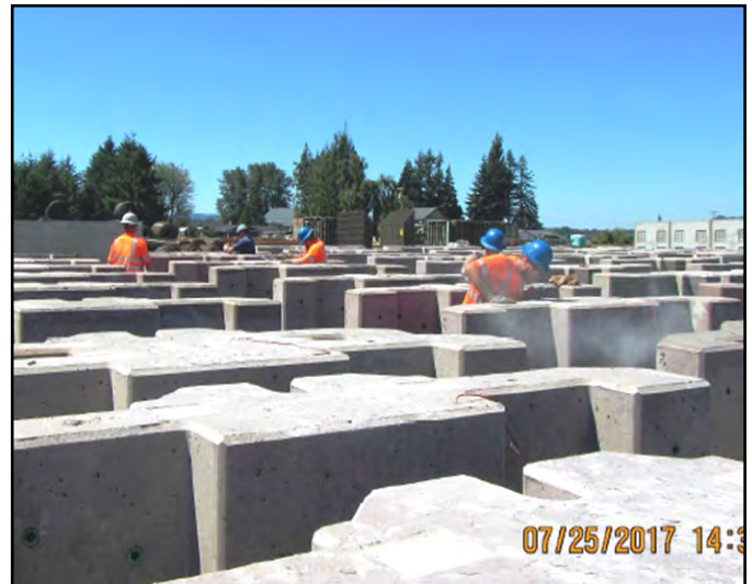
Columbia Precast: Crews performing minor concrete surface repairs.
