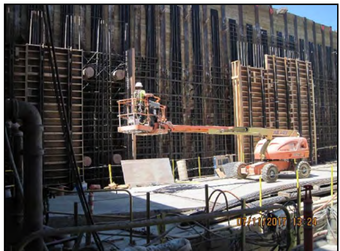
MLP: Installing rebar and formwork for the west portal wall.
