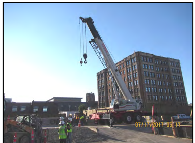
Mobilizing the 100-ton crane at the UDS.
