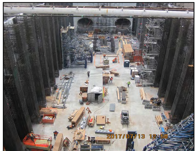
View of Roosevelt Station box looking south.
