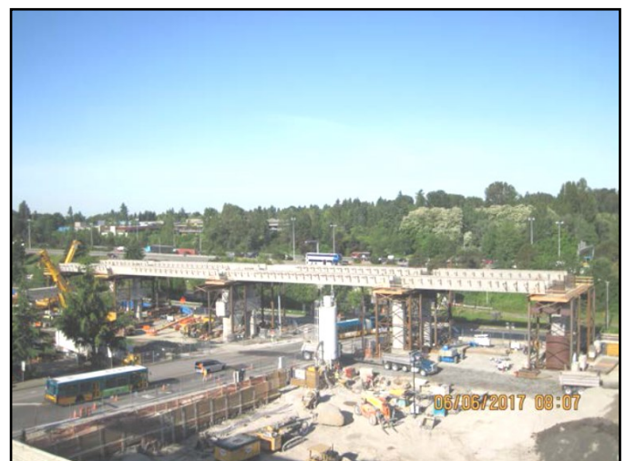
Girders placed from Bent C1 to Bent C5.
