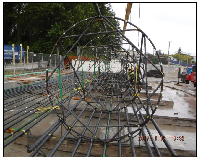
Assembling column cages to be used for drilled shaft.
