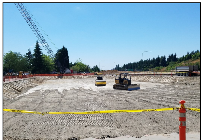
Excavation of OVS Infiltration Vault.
