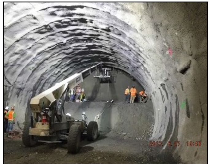
Installing lattice girder at top heading.
