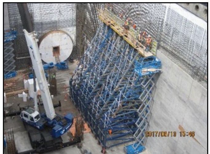
Setting the DOKA wall form for wall.
