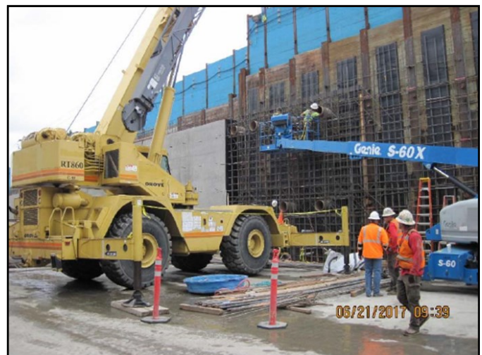
MLP: Installing rebar for east retaining wall before forming and concreting.
