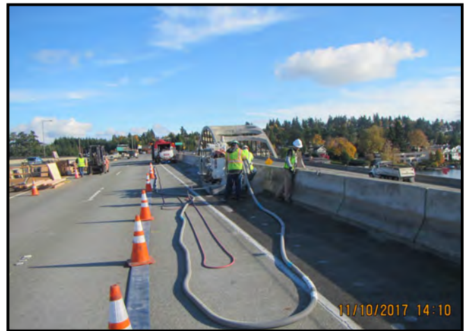
Removing south barrier at I-90.
