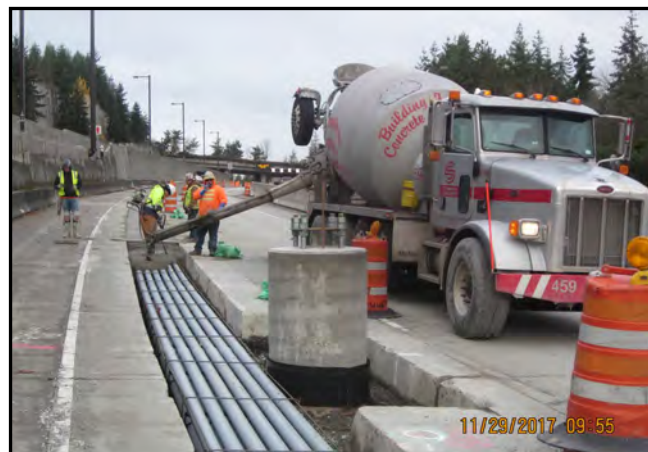
Systems duct bank installation ongoing.
