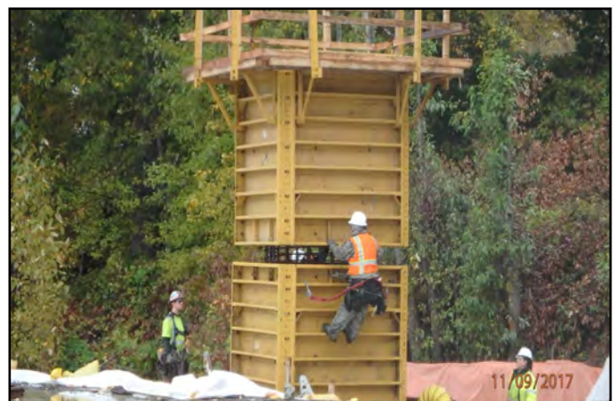
Setting of D11 column form.
