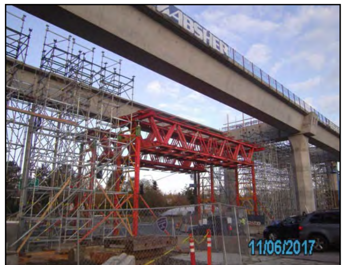
Absher Truss shoring crossing I03rd street
