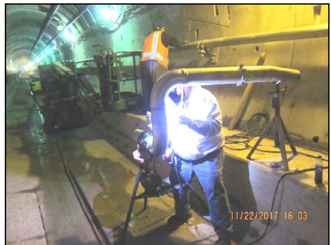
UDS-UWS: Welding fire standpipe tie-in section for CP37 SB tunnel.
