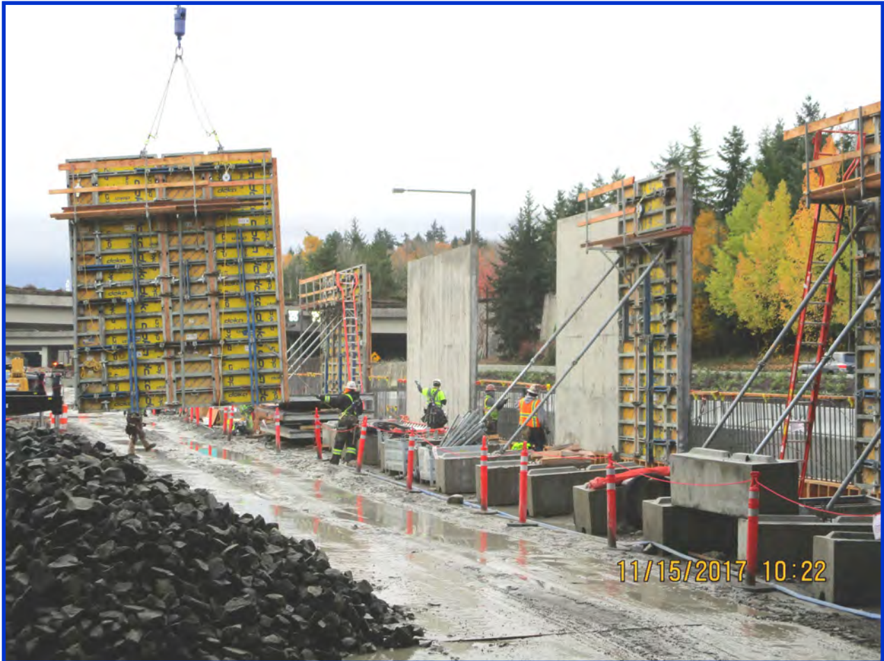
Setting Sound Wall Forms at Mercer Island Station (East Link Extension)
