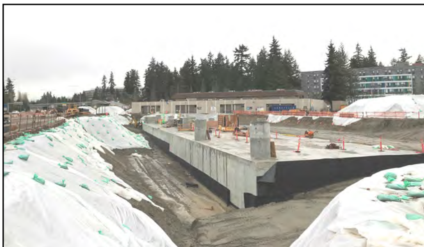
OVS Infiltration Vault CIP Wall Placement
