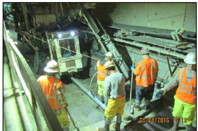
Lifting NB TBM No.1 cutterhead from the UWS shaft.
