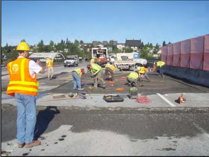
Installing loops prior to overlay of floating bridge.
