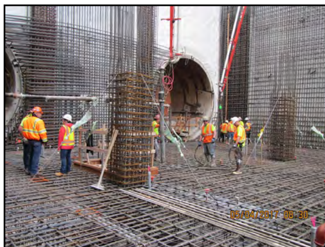
Preparing to place concrete for north pour 1.
