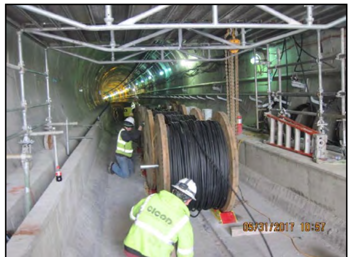
RVS to UDS: Pulling electrical wires in NB tunnel.
