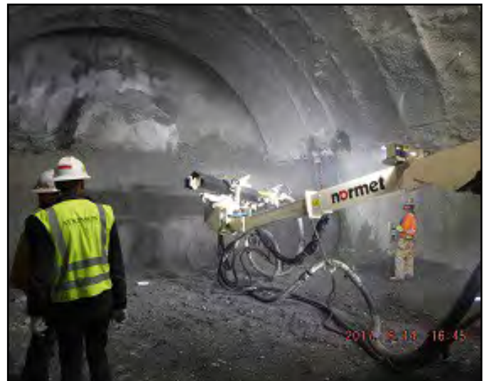
Installing shotcrete with new Normet robot for bench.
