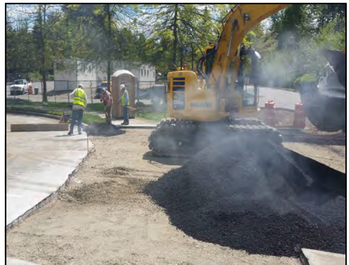
Crews prepping temporary OTC bus shuttle loop.
