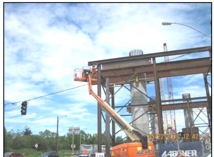
Welding girder support frame at Line C.
