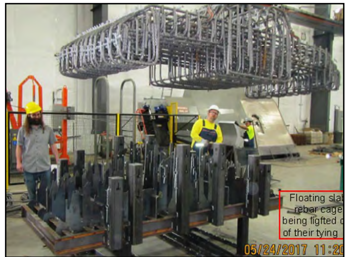
Floating slab rebar cage being lifted out of tying jig at CPP precast facility.
