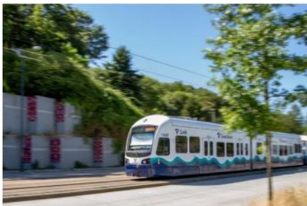
The Tacoma Dome Link Extension, scheduled to open in 2030, will add 9.7 miles of new rail between Federal Way and Tacoma. Photo courtesy of Sound Transit.
