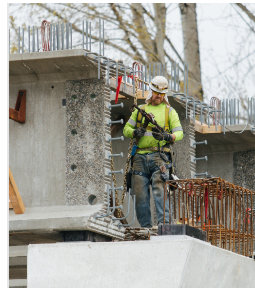
Constructing elevated guideway
