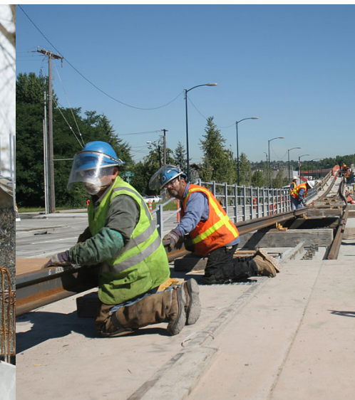
Laying light rail tracks
