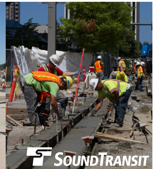
Restoring roadway and driveways
