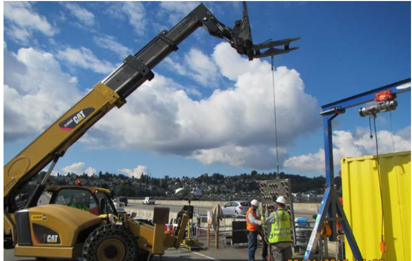
Crews lower a steel anchor cap into the floating bridge
