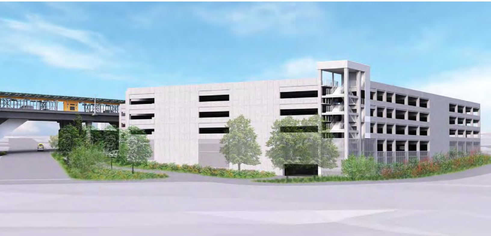
View of parking garage looking south
