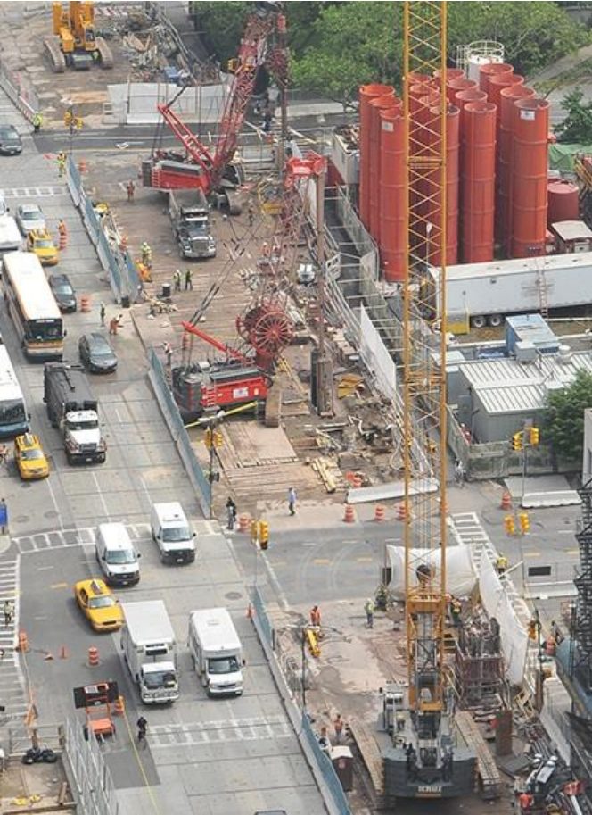
Cut and Cover Station Construction
