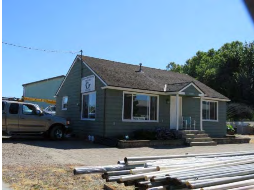
Figure 4-9. Gregory Drilling Office, Photographed on July 14, 2017, Facing Southwest
