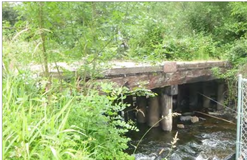
Figure 4-16. Bear Creek bridge, Photographed on June 27, 2017, Facing Northeast
