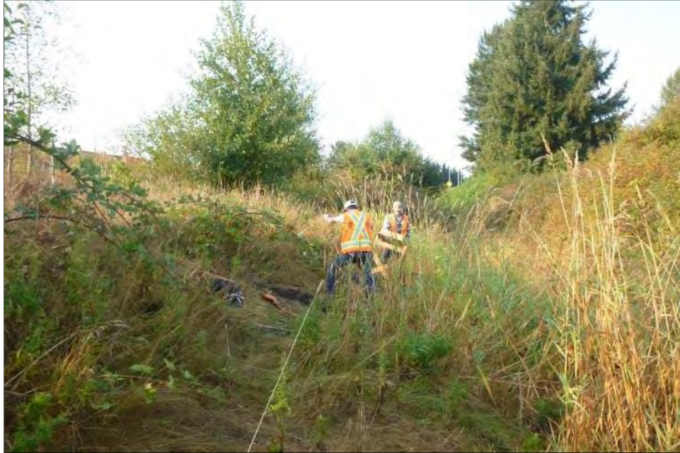
Figure 5-13. Ditch in WSDOT Right-of-Way in Area 2 Showing Auger 209 in Progress, Facing Southwest
