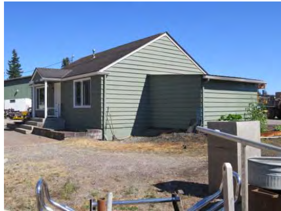
Gregory Drilling Office
