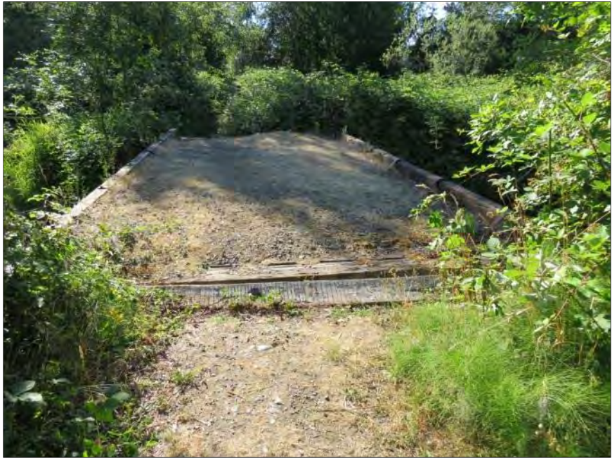
Figure 4-14. Bear Creek bridge, Photographed on July 14, 2017, Facing Northwest
