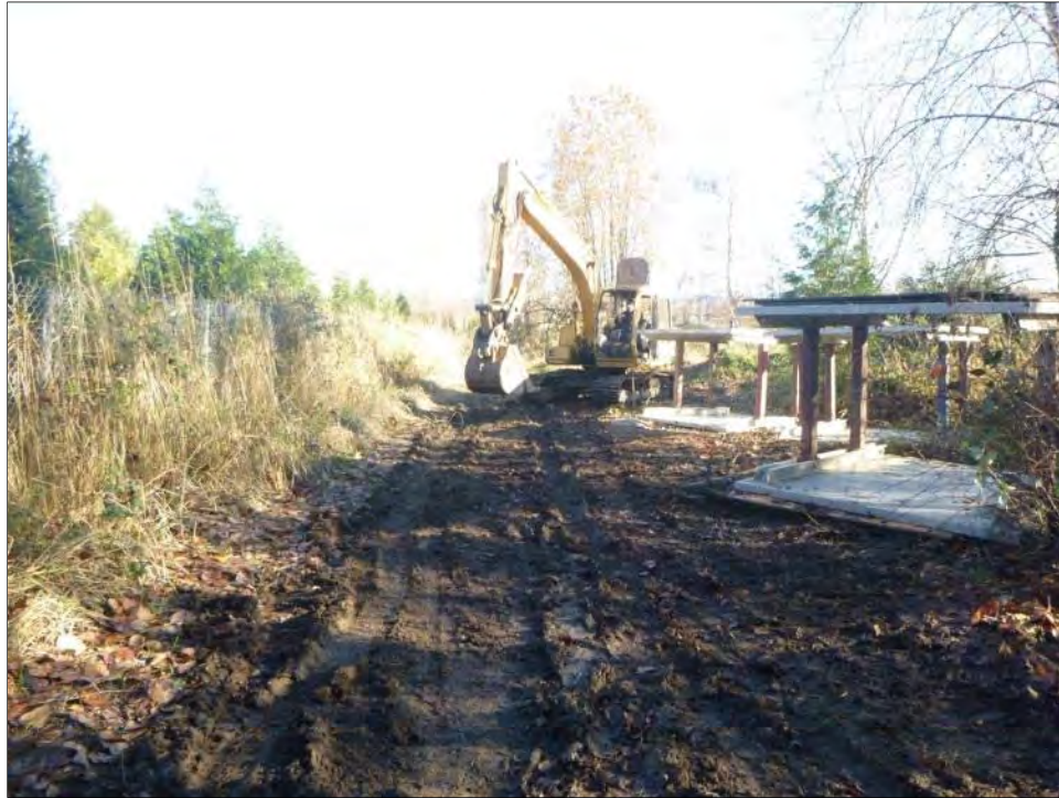
Figure 5-18. Location of Overburden Removal and Excavation Units Prior to Excavation, Facing East
