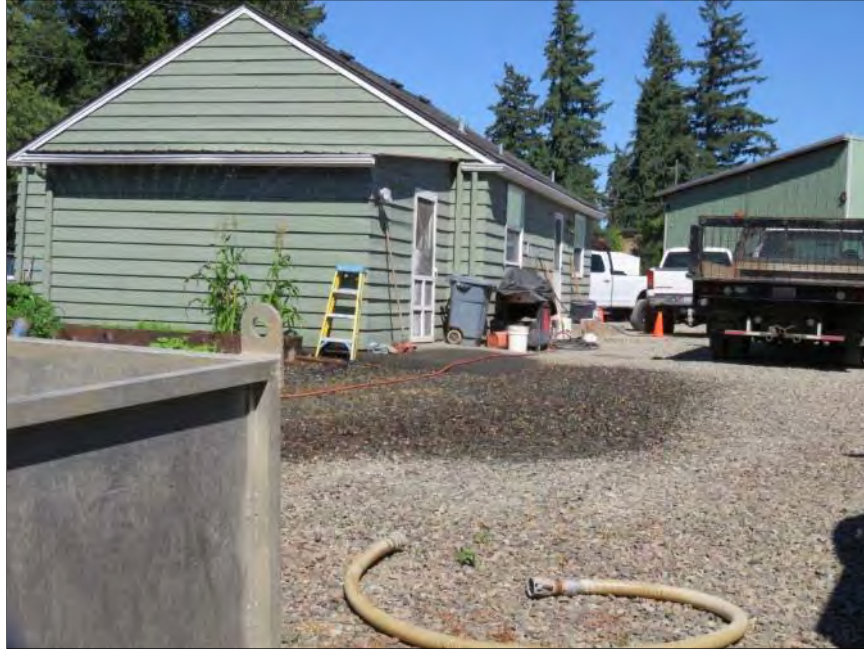
Figure 4-11. Gregory Drilling Office, Photographed on July 14, 2017, Facing East
