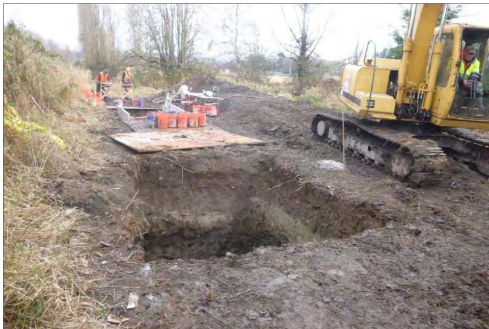
Figure 5-19. Trench 1 in Foreground and Trench 3 in Background, Facing East
