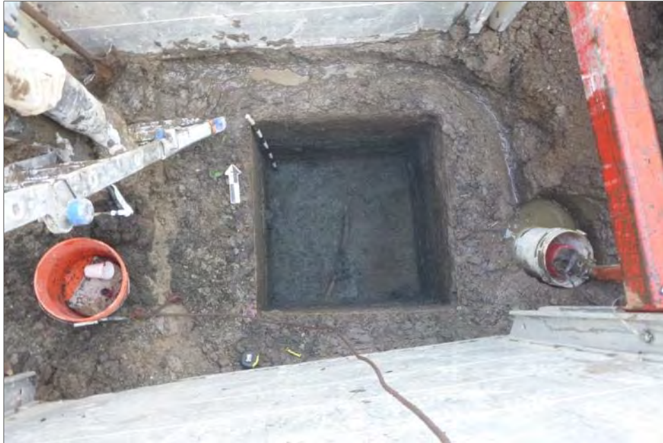
Figure 5-21. EU 1 in Trench 1 at 320 cmbd Prior to Extending Backhoe Excavation
