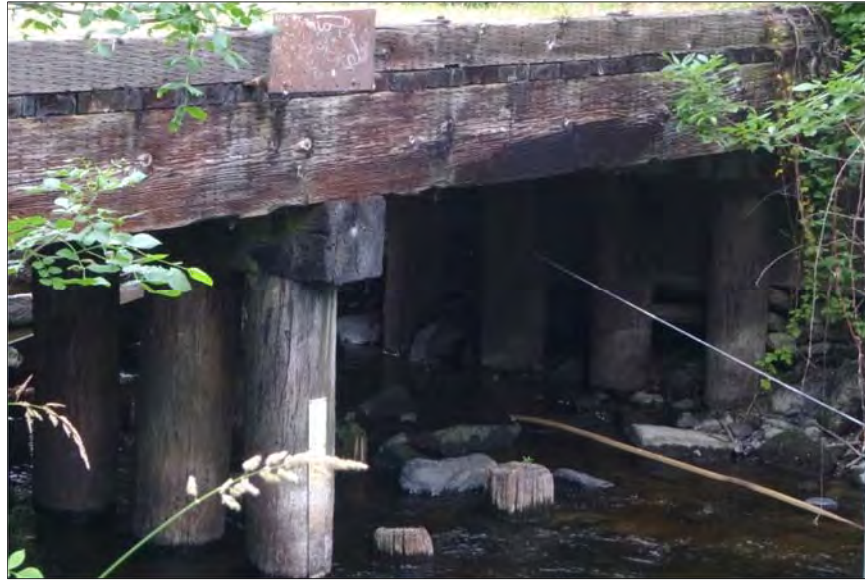
Figure 4-15. Bear Creek bridge, Photographed on June 27, 2017, Facing Northeast
