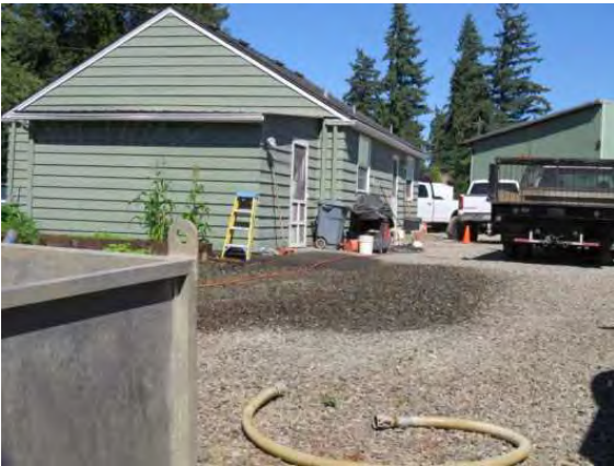
Gregory Drilling Office
