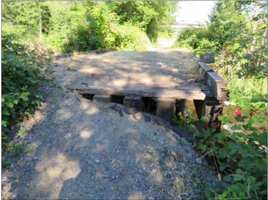
Figure 4-13. Bear Creek bridge, Photographed on July 14, 2017, Facing Southeast
