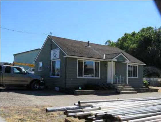
Gregory Drilling Office
