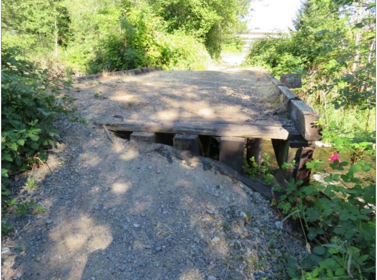
Existing Bear Creek bridge, facing southeast (Photographed on July 14, 2017)
