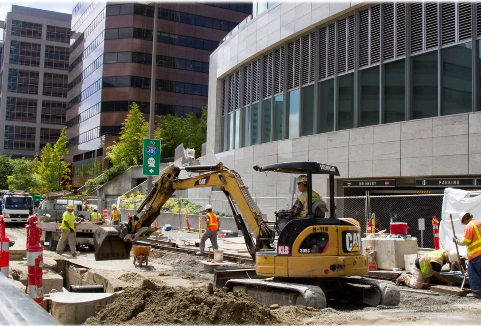
Downtown Bellevue north portal construction
