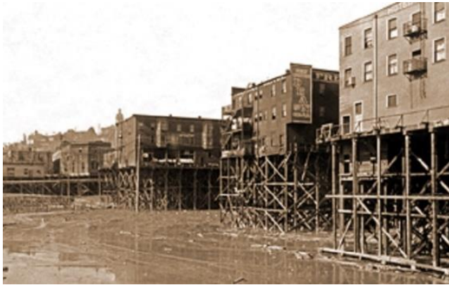
Fifth and Weller Streets in the Seattle Chinatown during the Jackson regrade c.1908.
