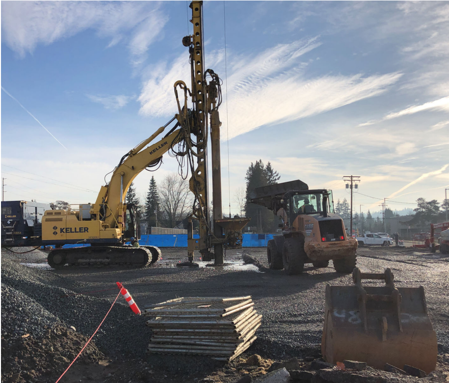
Installation of stone columns, ground improvements under garage & bridge
