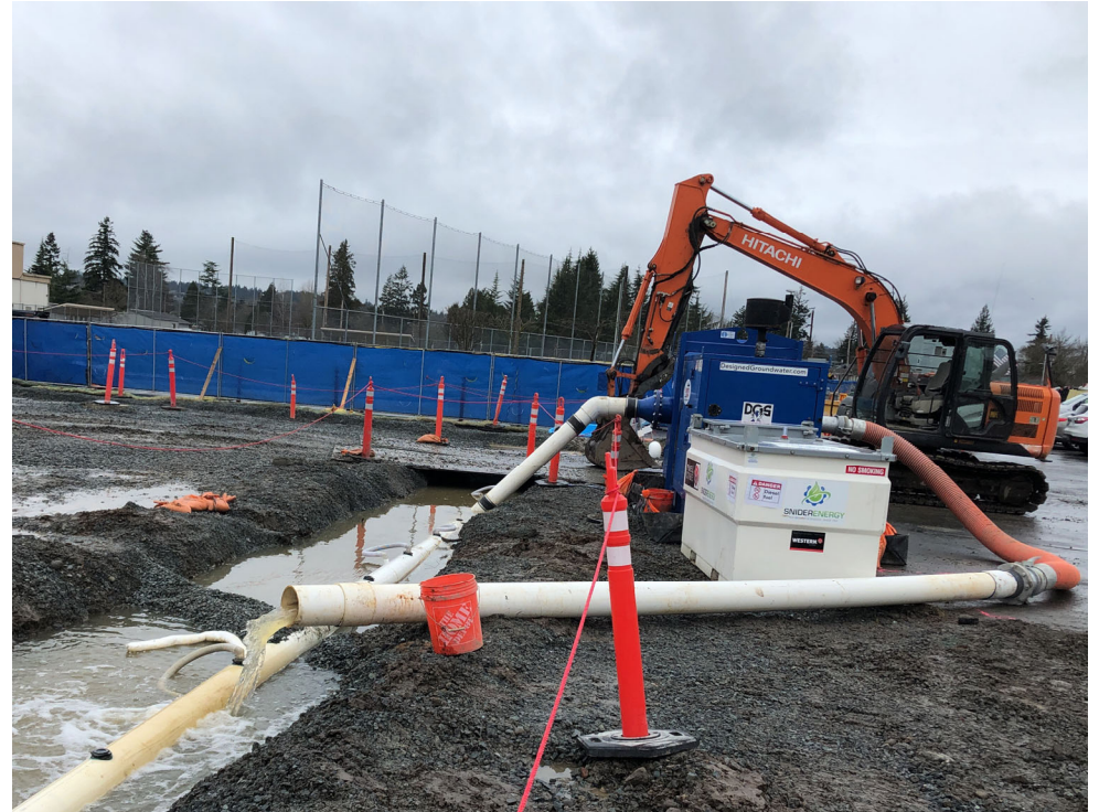
Installation of dewatering system around garage perimeter.
