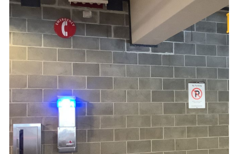
(NEW STANDARD EMERGENCY COMMUNICATIONS STATION)
